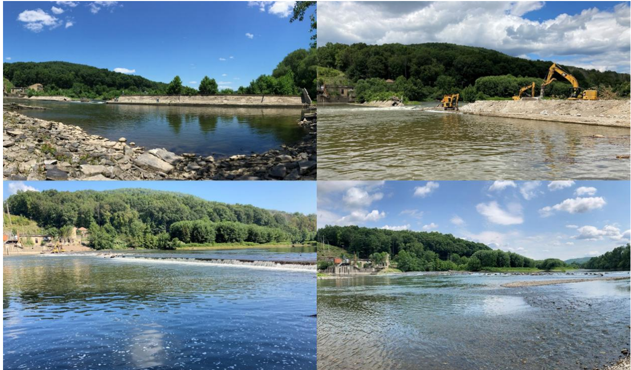
The Oakland Dam before, during, and after removal. This is the largest dam removal in Pennsylvania to date.
