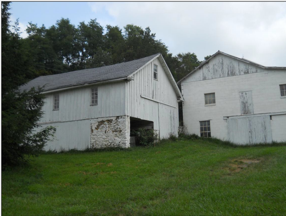
Wagon Shed, Lower Oxford Township, Chester County, c. 1880. Site 029-LO-002. This board and batten shed had ornamental trim on the cornices.
