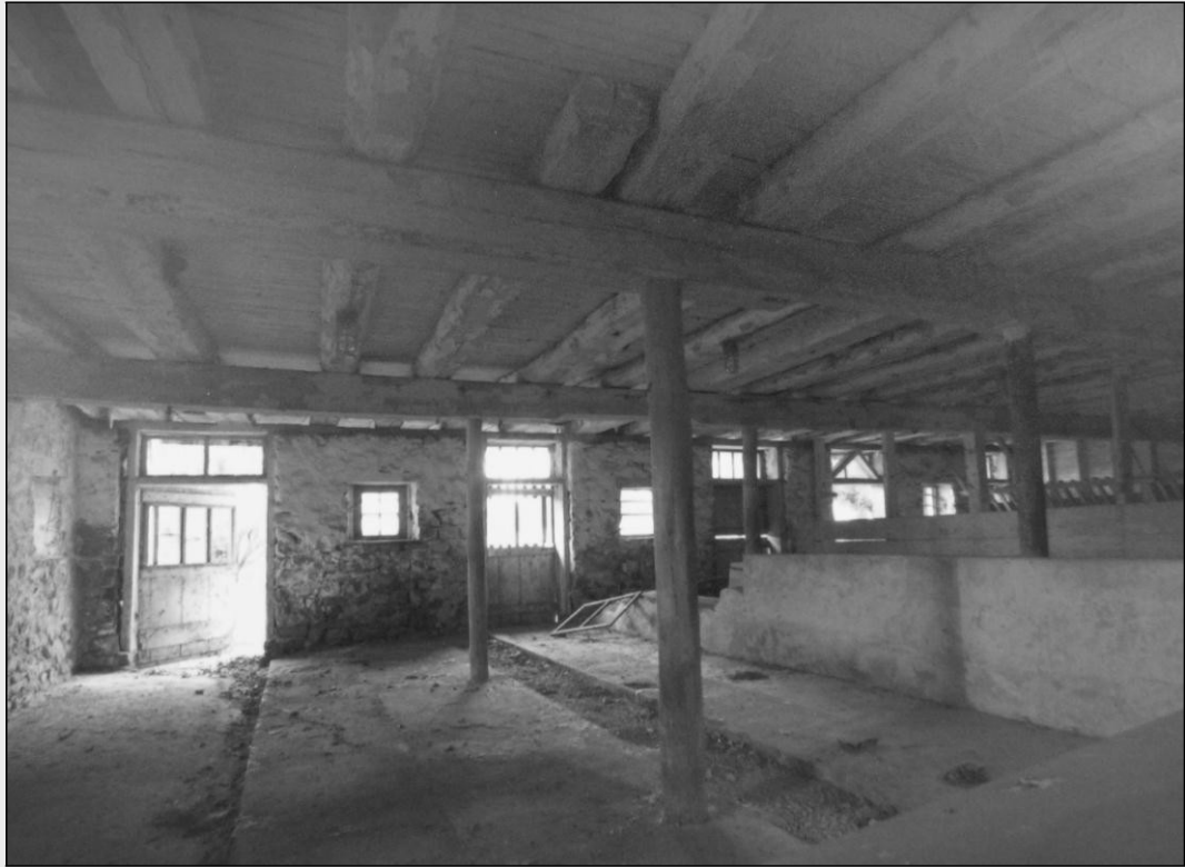
Barn interior showing 1930s – 40s installation of concrete floors, feeding troughs, and gutters to accommodate 20th C. dairy regulations. Rhoads-Lorah House and Barn, Amity Township, Berks County. Pennsylvania Historic Preservation Bureau file photo.
