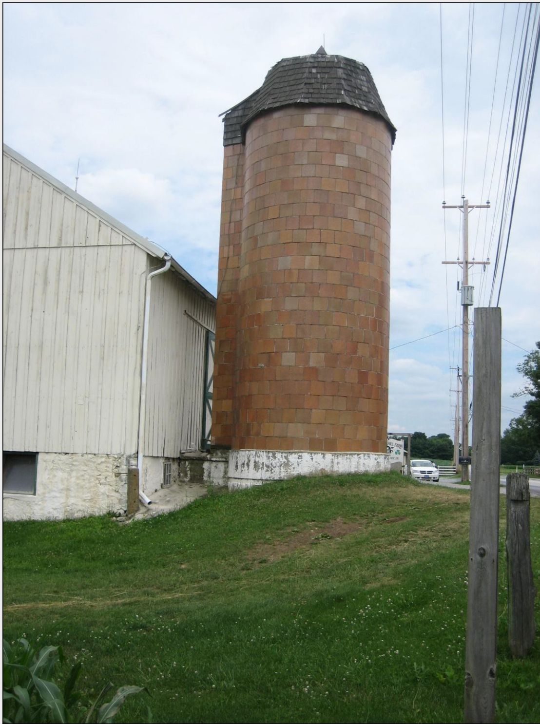
Tile silo with multi-sided shingle roof, West Brandywine Township, Chester County, c. 1930. Site 029-WB-001.
