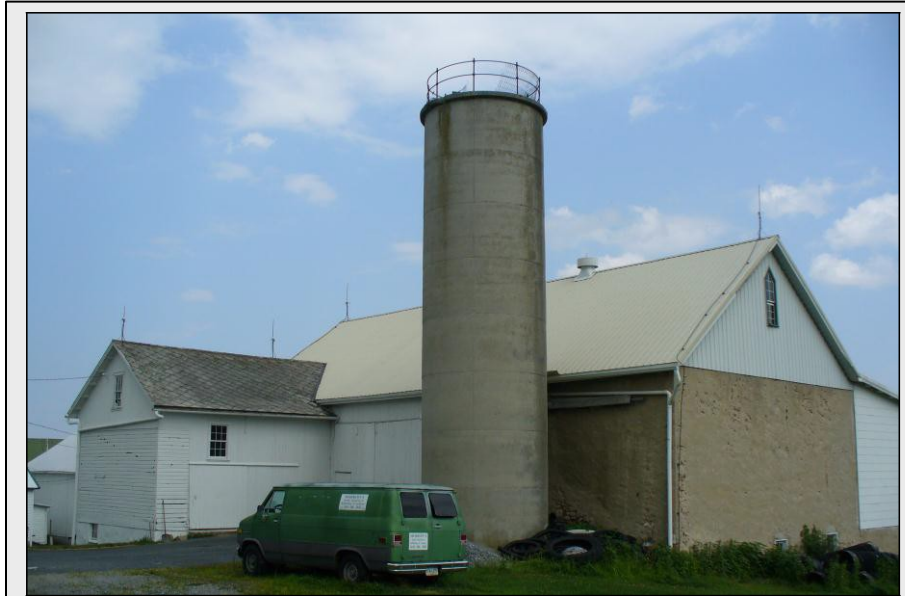
Poured concrete ring silo, c. 1950, West Nantmeal Township, Chester County. Site 029-WN-004
