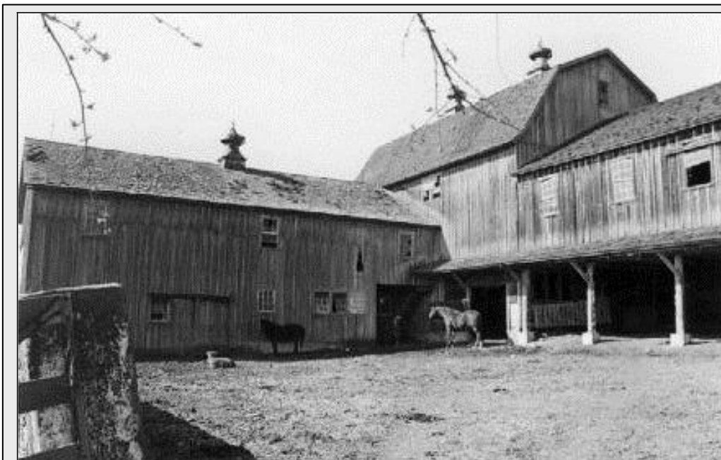
Pennsylvania Barn with ell extension off the forebay, Raven Hill Farm, Edgmont Township, Delaware County, date not given. Pennsylvania Historic Preservation Bureau file photo.
