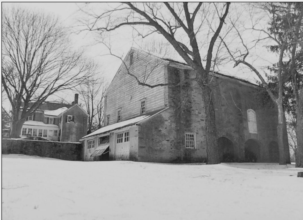
Pennsylvania Barn with stone arch forebay, Four-Way Farm, Springfield Township, Montgomery County, Early 19th century. Pennsylvania Historic Preservation Bureau file photo.
