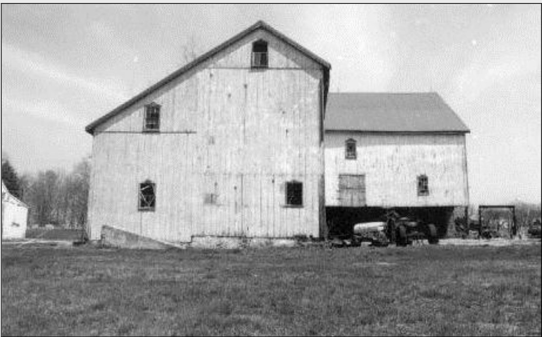
Forebay barn with two and one-half story ell addition and later shed addition, Humphrey-Eaton Farmstead, Montgomery Township, Montgomery County, no date given. Pennsylvania Historic Preservation Bureau file photo.
