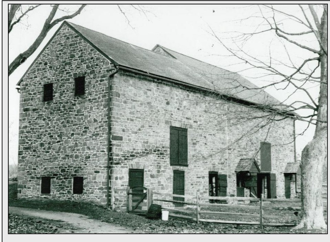
Front and rear elevations of "English Lake District" barn. The barn features a double ramp, and was constructed in two sections. The first portion (foreground) was constructed in 1796, and the larger section featuring a higher roofline was constructed in 1813. Isaiah Paxton Fann, Solebury Township, Bucks County. Pennsylvania Historic Preservation Bureau file.
