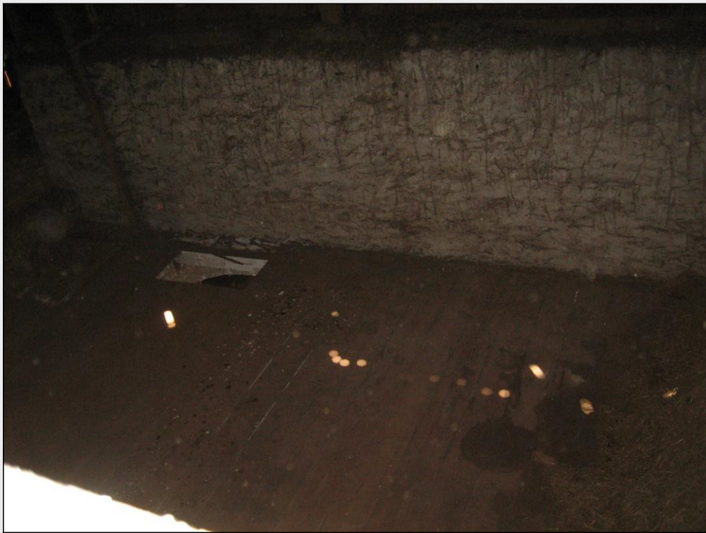
Double-decker barn, "sink mow" seen from threshing floor, West Bradford Township, Chester County, late 19th century. Site 029-WD-001. Note the opening in the floor for throwing hay down to the stables below.
