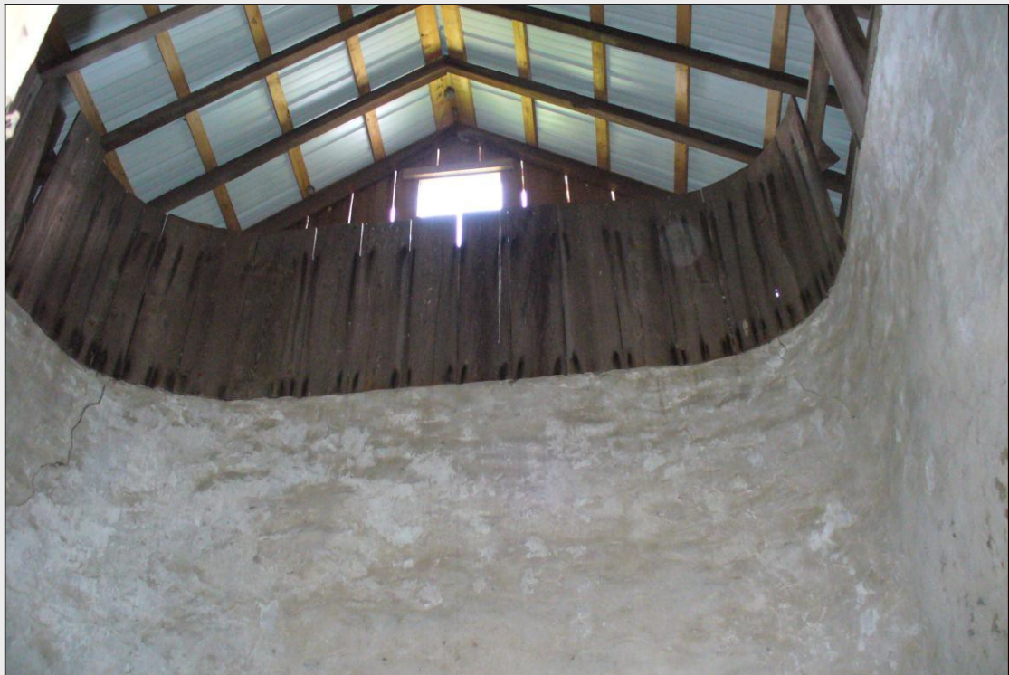
Interior view of the square stone silo depicted above. The corners are rounded, because farmers quickly discovered that silage got caught in square corners and was difficult to remove. Londonderry Township, Chester County.
