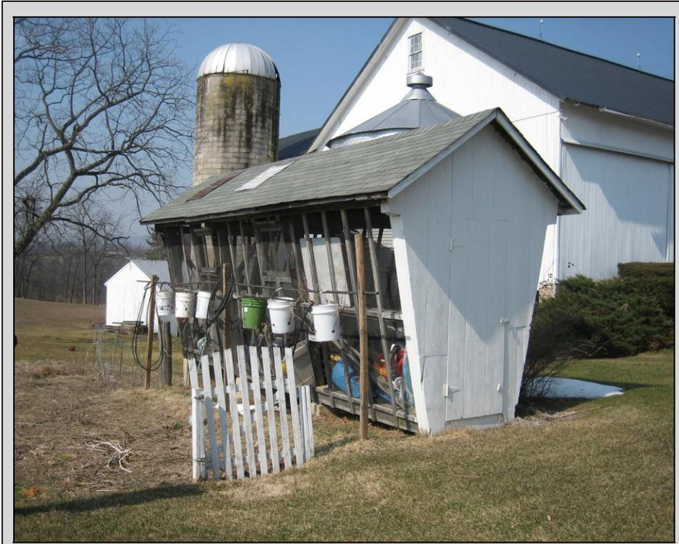
Corn Crib, Lynn Township, Lehigh County, c. 1950. Site 077-LY-002. This crib has the older style canted sides, but is built of modern materials including light wood frame and woven wire mesh sides. It is up on concrete blocks.
