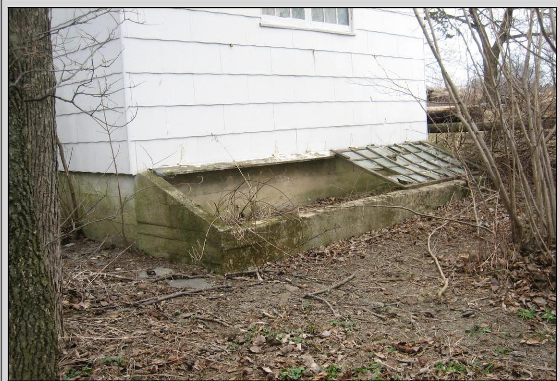
Cold frame, Lynn Township, Lehigh County, c. 1940-60. Site 077-LY-005. The frame would originally have been entirely covered with glass, which could probably be tilted partially open to admit cool air.
