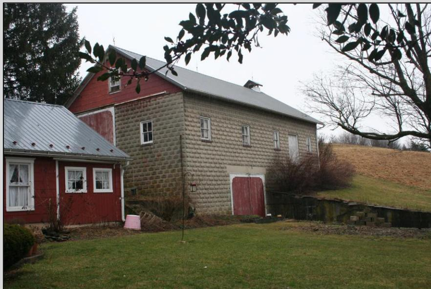
Potato barn, Heidelberg Township, Lehigh County, c. 1936. Site 077-HE-011. This fine cellar is built of rock-face concrete block and has access on the upper level gable and eaves. Reportedly the earth fill for the bank was obtained when the road was widened in the 1930s by a New Deal public works project.
