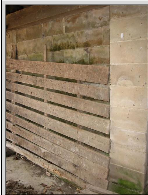
Potato barn lower level interior showing wood slats attached to masonry walls, Lynn Township, Lehigh County, c. 1935-50. Site 077-LY-004.
