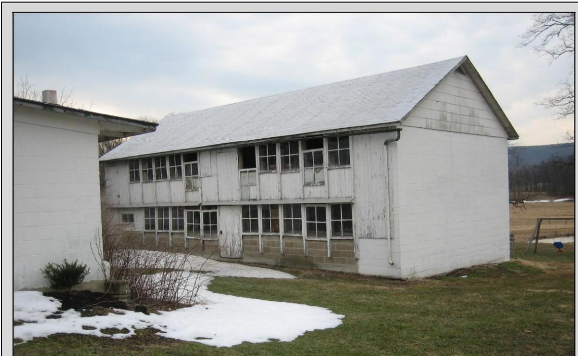
Poultry house, Heidelberg Township, Lehigh County, c. 1960. Site 077-HE-002. This building had a brooder house inside it with chimney for the stove pipe that heated the brooder area.
