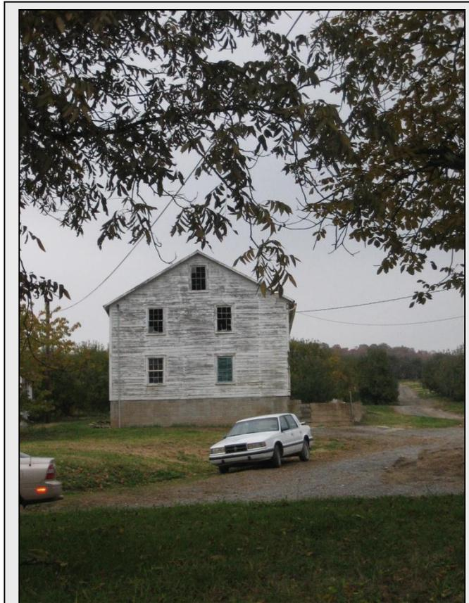
Packing House, Menallen Township, Adams County, c. 1930-50. Site 001-ME-005. This two story building has a concrete block foundation. The ample lighting and eaves-side garage style doors that indicate that packing was done here.
