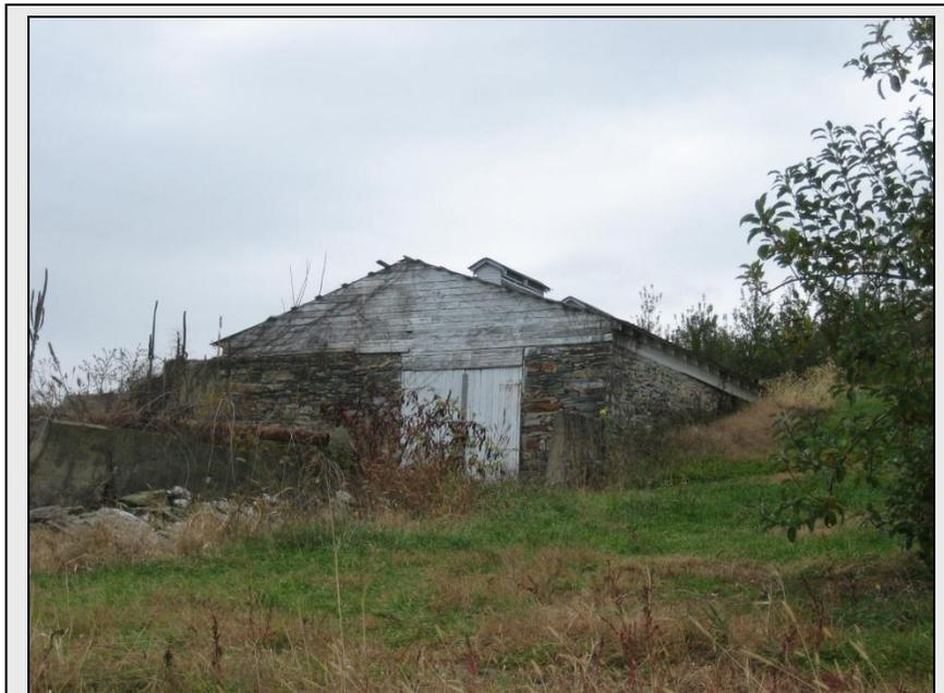
Farm cold storage, Huntington Township, Adams County, early 20th century. Site 001-HU-003. Note the characteristic features of "common" cold storage: roof ridge ventilators, banked construction, thick walls of good insulating material (in this case, stone masonry), and sliding doors at grade for easy loading.
