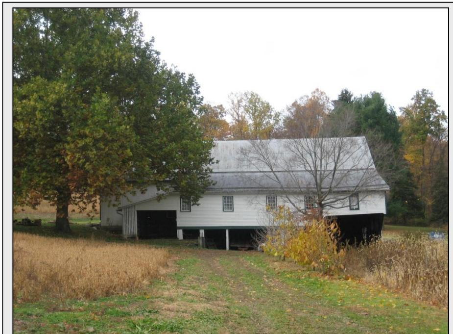
Forebay barn with shed-roof addition possibly used for packing. The windows are larger and more carefully finished than poultry windows would be. Menallen Township, Adams County, barn c. 1880, alteration c. 1940. Site 001-ME-004.
