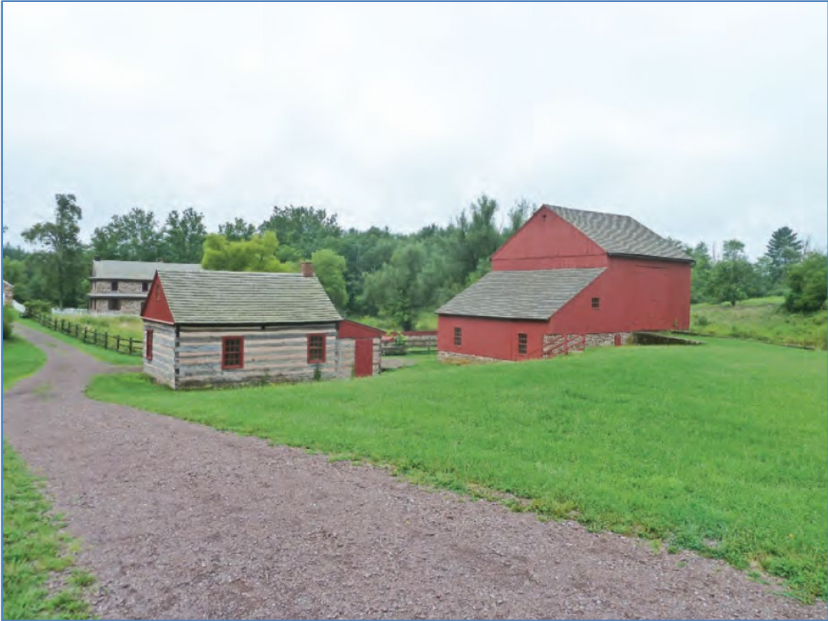
Figure 5: Homestead Barn (right) and blacksmith shop (left) with Daniel Boone House in the distance.
