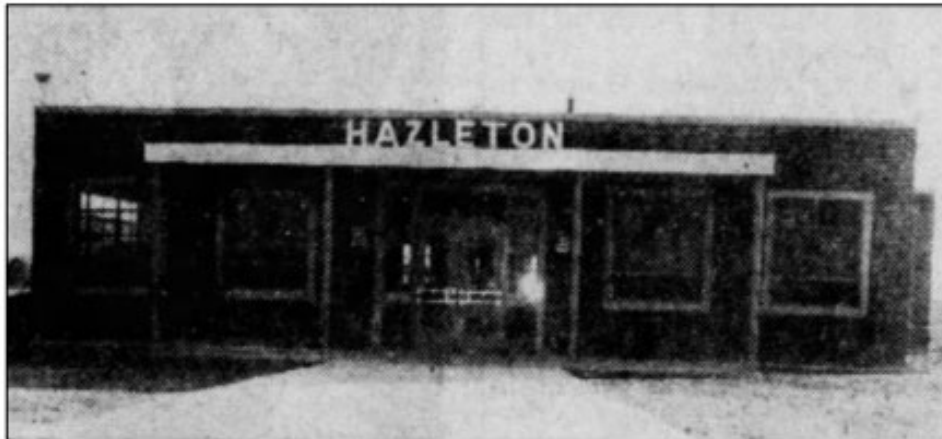
Figure 4: 1953 Photograph of northern (street side) façade of terminal (MB-13), from November 6, 1953 article in the Plain Speaker , facing south.
