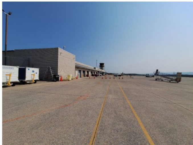
Photo 15: Southwest (far left) and southeast (center) elevations of the Terminal Building, showing the apron, view northeast.
