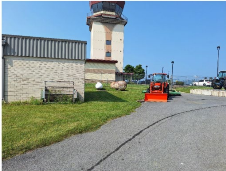
Photo 1: Northwest end of the Terminal Building at left, with Air Traffic Control Tower (ATCT) at center, view west.
