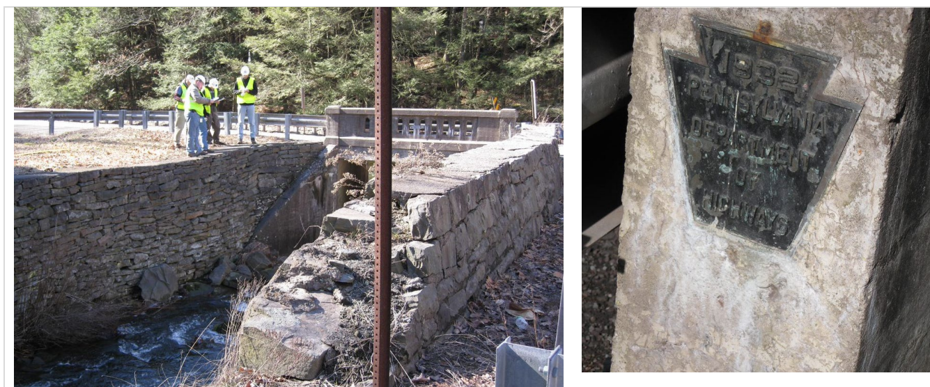
Photographs 31 and 32. Adjacent and connected concrete bridge on State Route 29, Luzerne County. Note DOH 1932 keystone plaque showing both WPA & DOH involvement with same resource. Potentially eligible given size and scale, workmanship, and documented WPA association. All photos from PennDOT. The bridge, previously unevaluated, contributes to this planned landscape.
