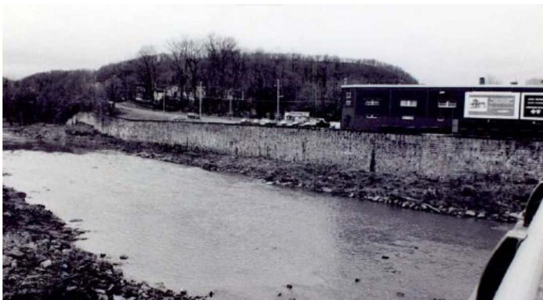
Photograph 12. Channelized stream WPA masonry wall (1936), 301 Central Avenue, Johnstown, Cambia County. Resource # 1995RE46944. This section is 925' in length and is the only remaining portion of stone wall not covered with concrete. Photo from PA SHPO files. Mapped and determined National Register eligible in 1995 as part of Johnstown flood protection system along the left bank of the Stonycreek River.
