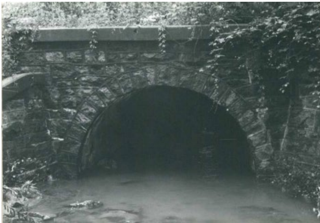
Photograph 16. WPA era culvert (1940) on State Route 61 over Mud Run, Ryan Township, Schuylkill County. Resource # 2002RE02925. Photo from PA SHPO files. Mapped and determined not eligible in 2016 due to loss of integrity associated with removal of stone on opposite elevation.
