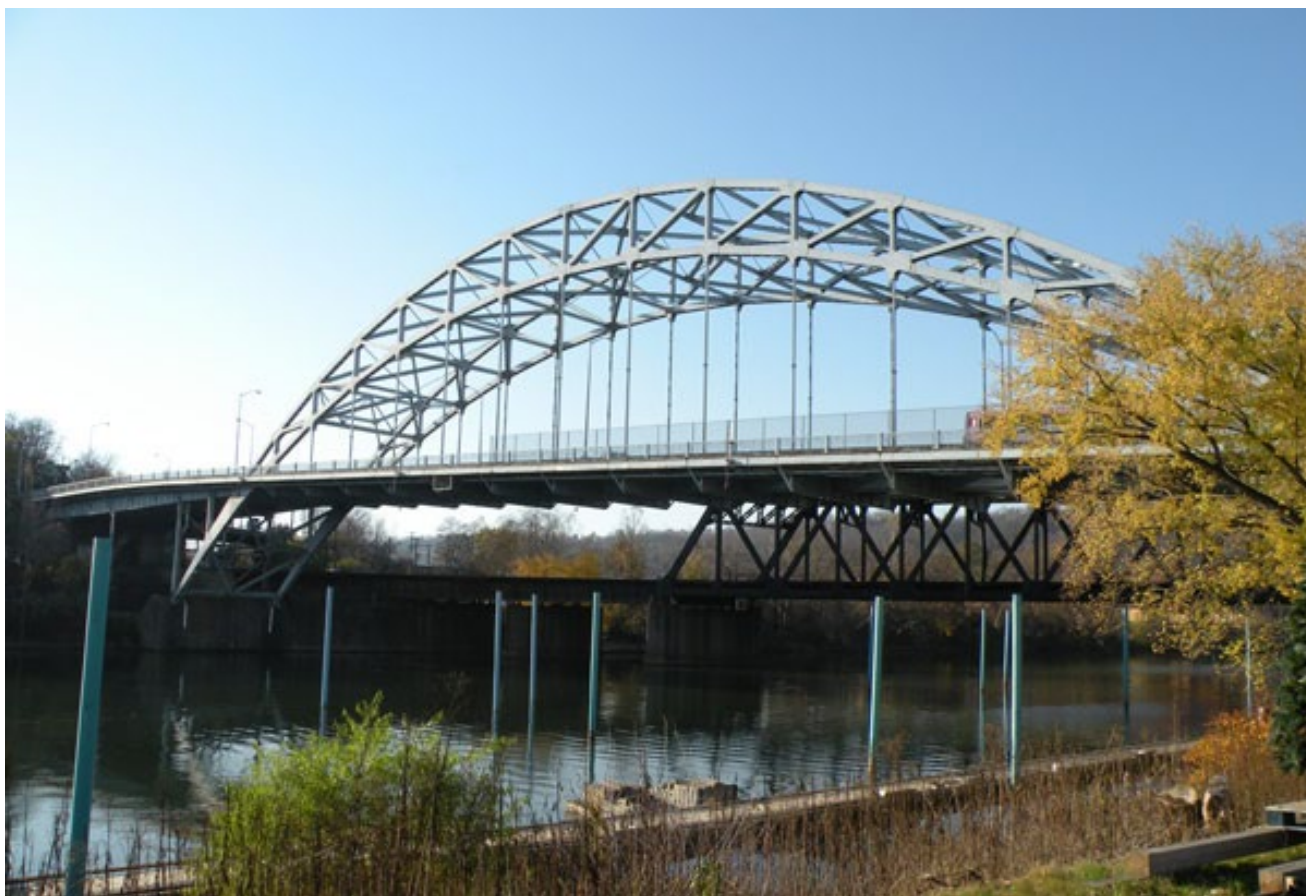
Photograph 4. Jerome Street Bridge (1939), LR 392, McKeesport, Westmoreland County. Resource # 1986RE00922. Significant for engineering as a two hinged through arch bridge. CCC involvement not noted in National Register listing. Photo from livingnewdeal.org. Mapped and National Register listed in 1986.
