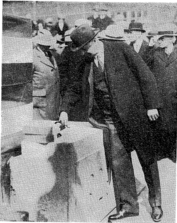
Governor Fisher Lays Cornerstone of Main Building—1930.
