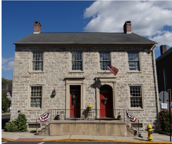
This prominent house on Chestnut Street was built by Jacob Vogel in 1813. It is an excellent example of an early Federal-style residence and retains distinctive characteristics like limestone walls, chimneys at the gable walls, two doors with simple wood trim, and large wood windows divided into 12 small panes of glass.
