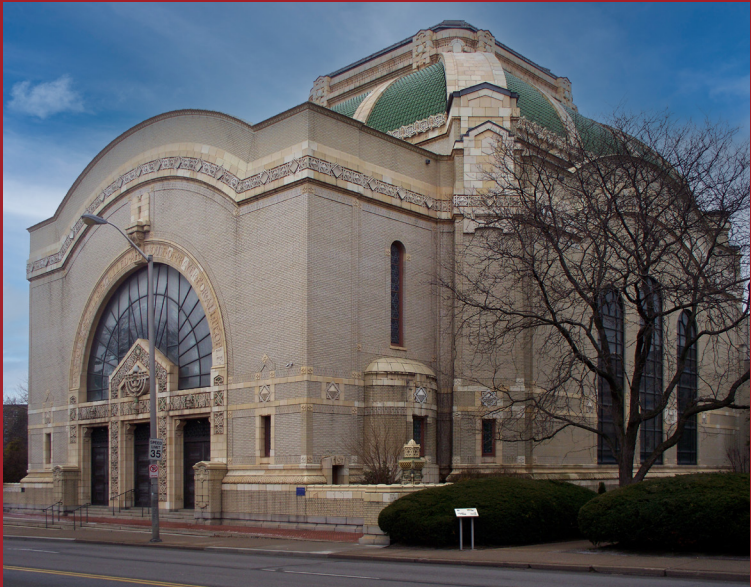
The statewide plan educational meeting and listening session in Pittsburgh was held at Temple Rodef Shalom. This home of the Rodef Shalom Congregation was designed by architect Henry Hornbostel in 1906 and was listed in the National Register of Historic Places in 1979.
