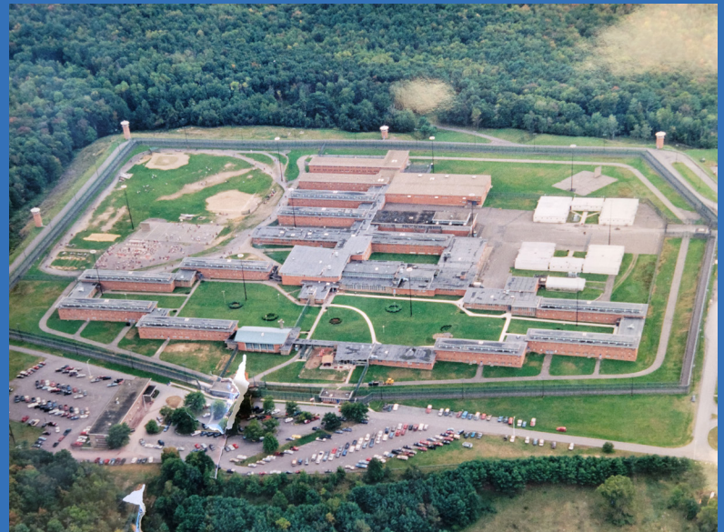
A collection of more than 50 buildings and structures on over 1,000 acres in Luzerne County, SCI Dallas is important as a state correctional institution for young adults and for its collection of International Style buildings utilizing plans popular for correctional institutions in the mid-20th century.
