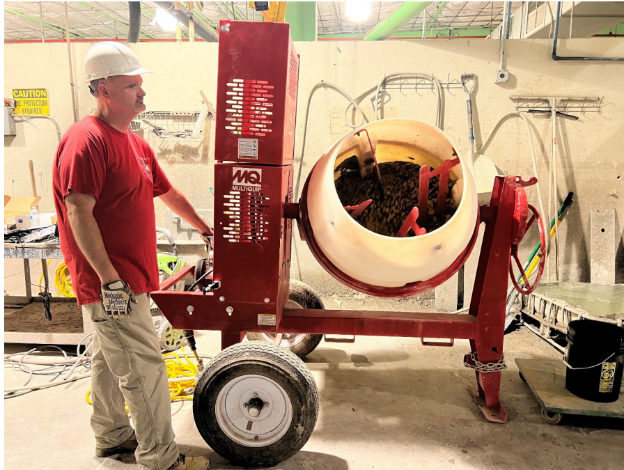
Figure 41. Uniform blending water and aggregate inside the mixer.
