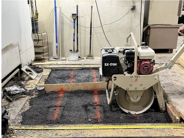
Figure 29. A roller compactor was used in this study.
