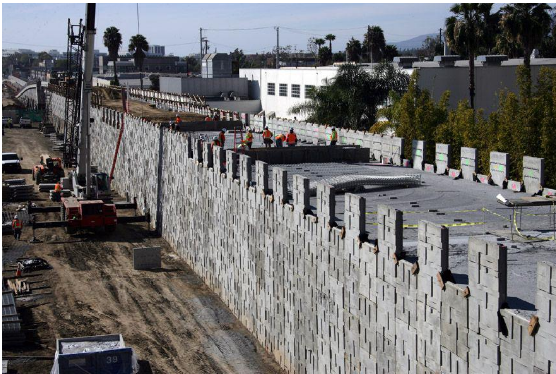
Figure 1.7. LCC backfill for an MSE wall light rail project in California (Schaefer et al. 2017a).
