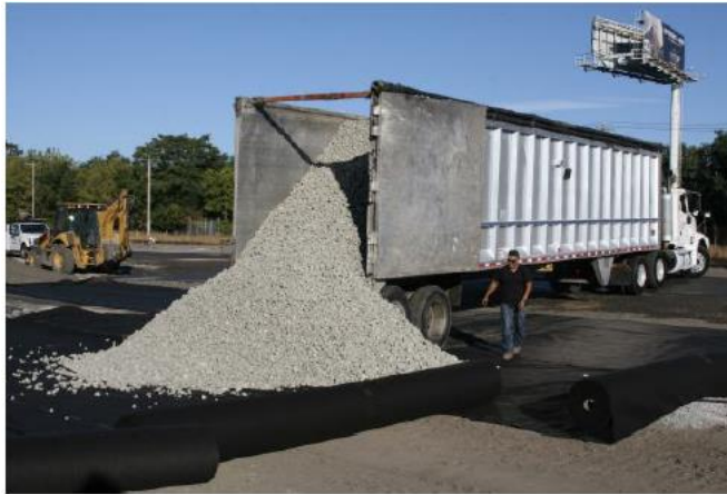
Figure 4.41. Delivery and unloading of FGA.
