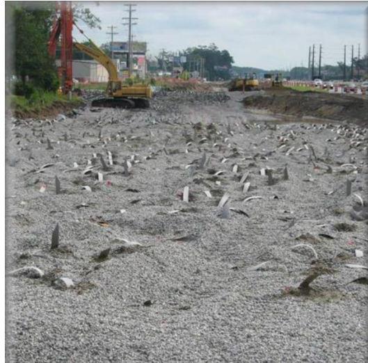
Figure 4.34. Installation of vertical drain for embankment cases.
