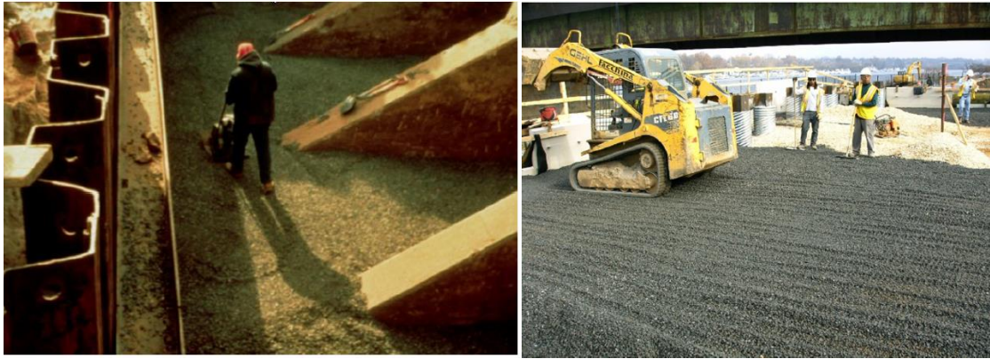
Figure 4.37. Vibratory plate compactor (Left) and hauling dozers (Right) for ESCS placement.
