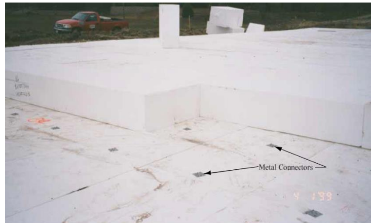
Figure 4.25. Photo showing arrangement of EPS blocks and placement of mechanical connectors (Virginia Department of Transportation).
