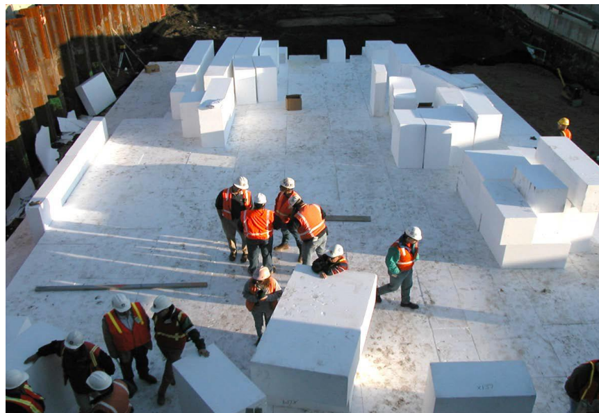
Figure 1.2. EPS-block geofoam used for embankment construction (Schaefer et al. 2017a).
