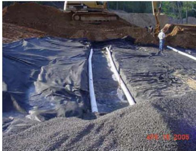
Figure 4.18. Placement of pipe drains to divert water away from the area where EPS-block Geofoam is to be placed (Alabama Department of Transportation).
