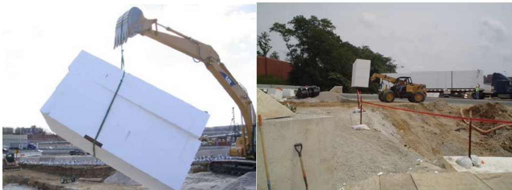
Figure 4.20. (a) Using a trackhoe to move EPS blocks and putting structural steel angles to protect bottom edges of blocks from damage due to straps. The top edges of the blocks are unprotected (Virginia Department of Transportation) (b) Moving EPS blocks to storage area using a forklift (Virginia Department of Transportation).
