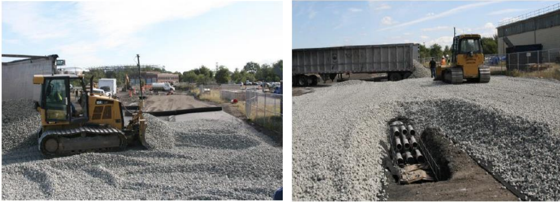
Figure 4.42. Placement and compaction of FGA.
