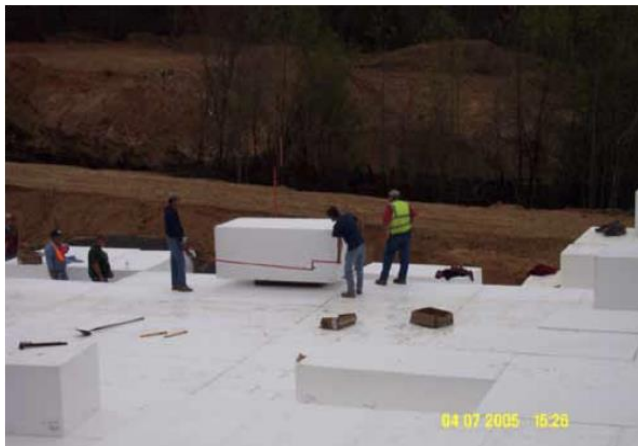
Figure 4.23. EPS block installation: (a) Placement crews lifting and moving EPS blocks using gripper (Alabama Department of Transportation); (b) use of a scissor clamp to place blocks as part of the new Topaz Bridge project in Idaho (Horvath).
