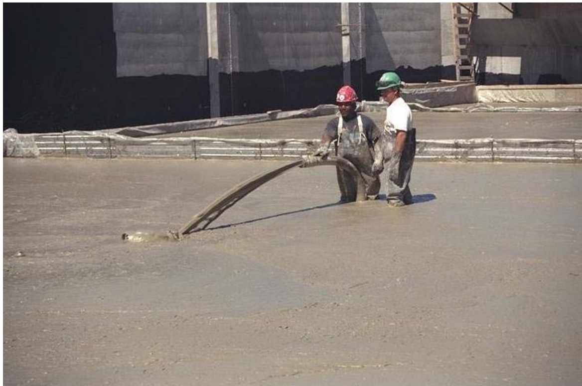
Figure 1.9. On-site production and placement of LCC (courtesy of Aerix Industries TM ).
