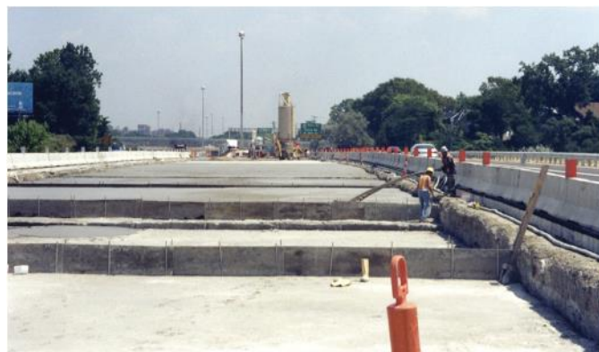
Figure 4.31. Placement of separated LCC lifts.
