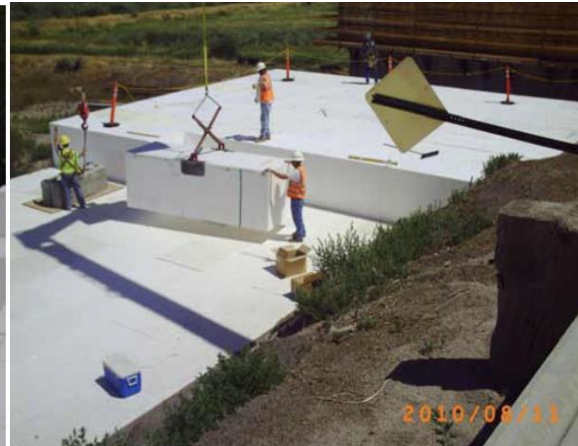
Figure 4.23. EPS block installation: (a) Placement crews lifting and moving EPS blocks using gripper (Alabama Department of Transportation); (b) use of a scissor clamp to place blocks as part of the new Topaz Bridge project in Idaho (Horvath).
