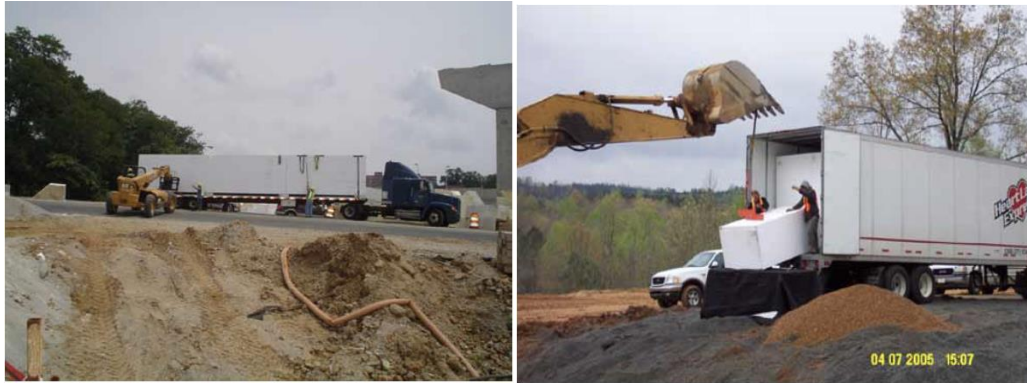
Figure 4.19. (a) Unloading EPS blocks from open flat-bed trailer upon arrival at job site (Virginia Department of Transportation) (b) Unloading EPS blocks from closed upon arrival on site (Alabama Department of Transportation).
