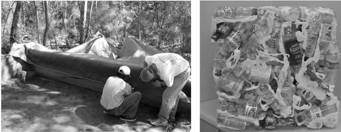
Figure 1.39. Graettinger et al. (2005) case history: (Left) attaching woven geotextile to retaining wall; (Left) laboratory sample of lightweight fill composed of recycled plastics.
