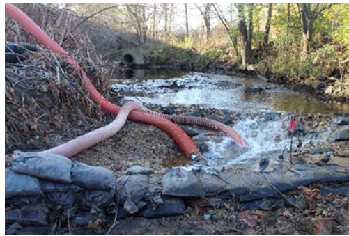
Photo 17a Upstream Cofferdam
