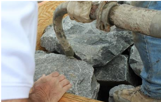
Photo 11 Elbow Tube Used to Deliver Grout
