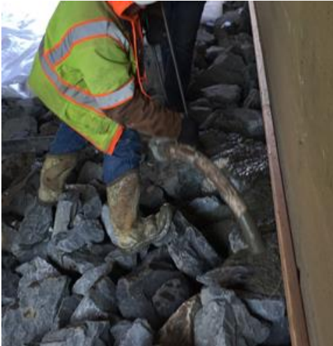
Photo 31 Grout Placement at Interface
