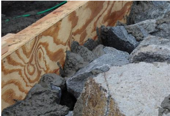
Photo 9 Grout Alongside the Form Wall
