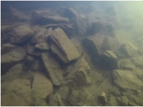
Photo 39 Under Water View of PGR at Abutment side
