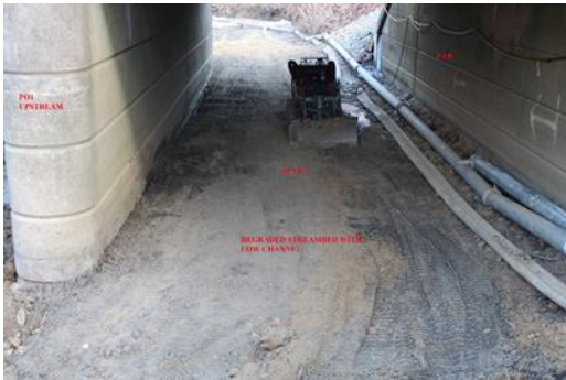
Photo 33 Regraded Streambed with Low Channel in Span 2
