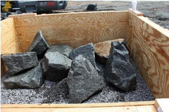
Photo 7 Placement of Rocks
