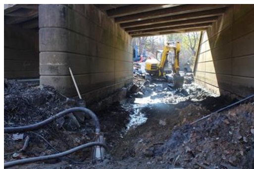
Photo 24 Removal of Existing Rocks in Span 1
