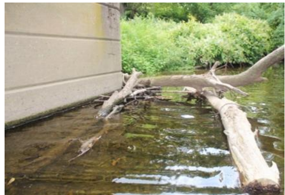
Photo 45 Debris at Upstream of Pier Nose and Span 1
