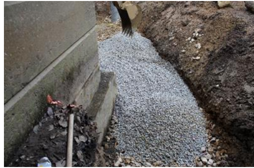
Photo 26 Placing 2-inch of AASHTO No 57 to Level Base
