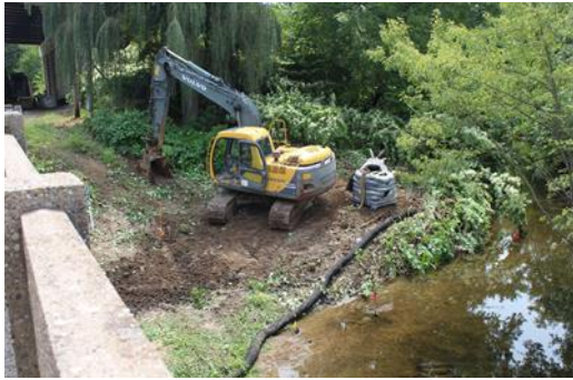
Photo 16 Upstream Construction Entrance
