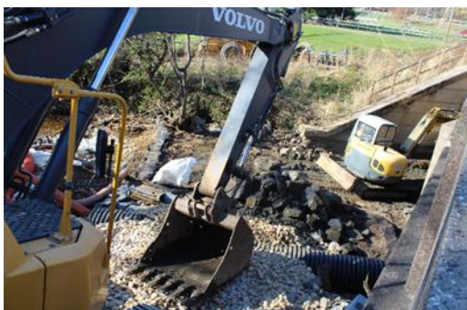
Photo 23 Large and Mini Track Excavators
