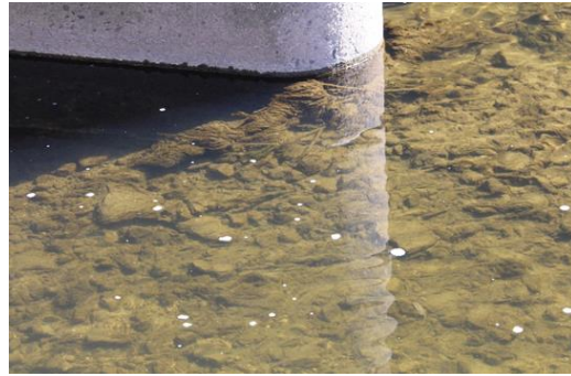
Photo 42 Filamentous Algae Growth on Top of PGR
