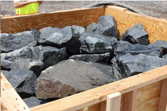
Photo 8 Final Rock Placement in the Form
