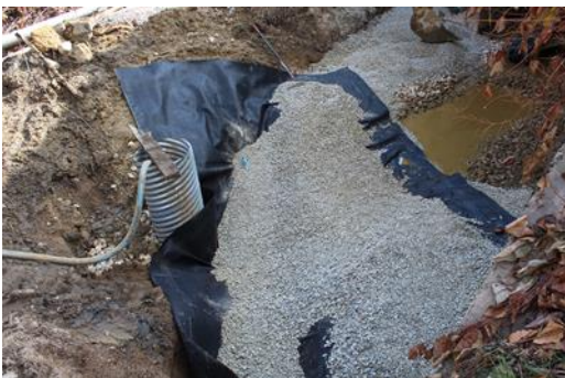
Photo 27 Placement of Combined Filter
