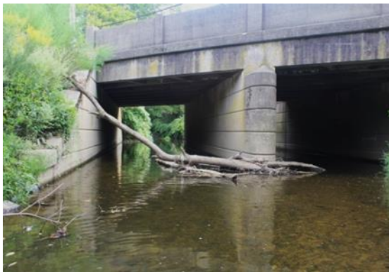
Photo 45 Debris at Upstream of Pier Nose and Span 1
