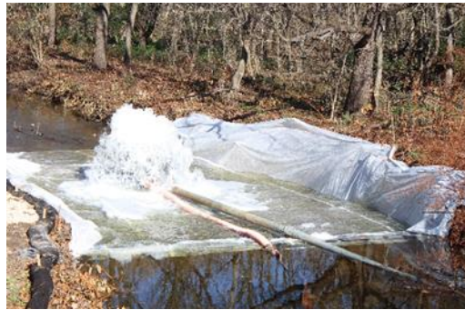
Photo 18 Downstream Energy Dissipater
