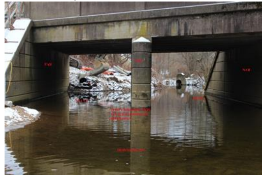
Photo 32 6-inches of Streambed Material Placed on Top of PGR
