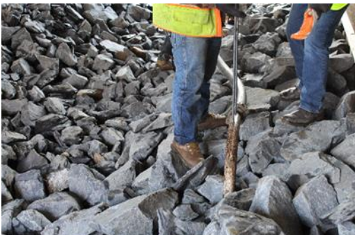
Photo 29: Modified Grout End Delivery
