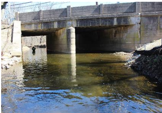
First On-Site Inspection
