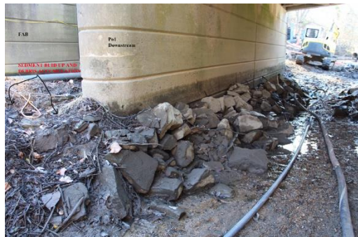
Photo 22 Preconstruction Condition of Span 1
