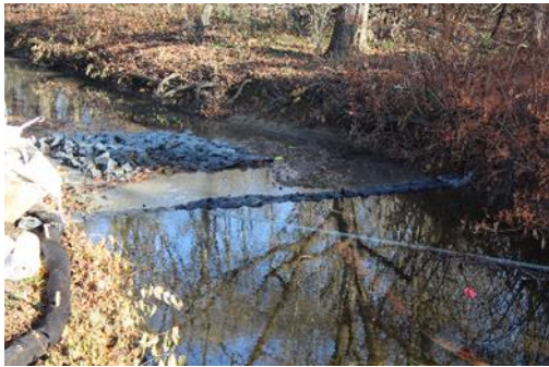
Photo 17b Downstream Cofferdam
