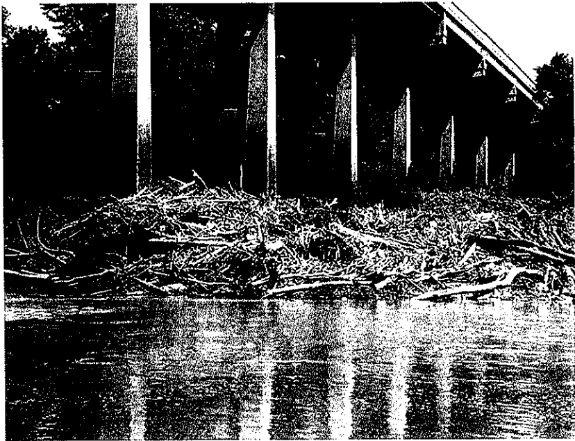
DRIFT AT BENT #8, TYPICAL
