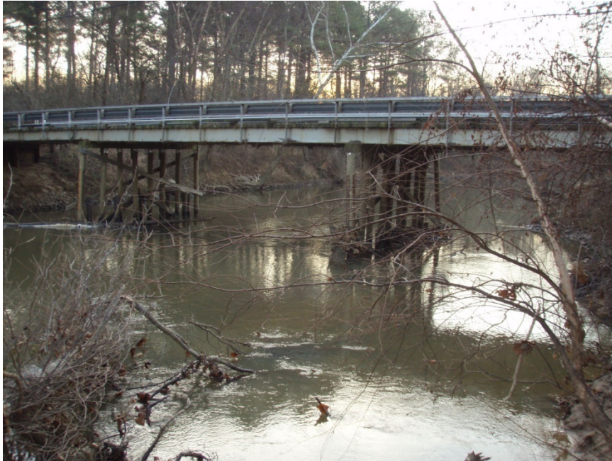
Figure 17. VA 716 bridge over the Banister River, Halifax Co., VA.
