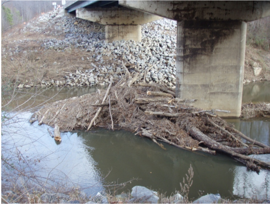
Figure 21. VA 138 bridge over the Mehrrin River, Lunenburg/Mecklenburg Co. line, VA.
