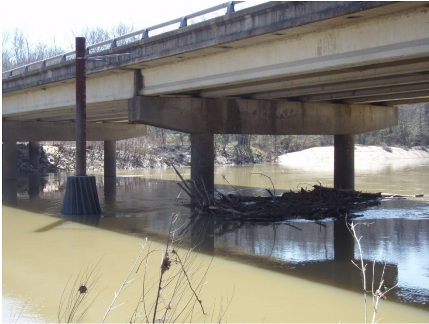
Figure 27. TN 005 (US Rt. 45) over the Obion River, Obion Co., TN.
