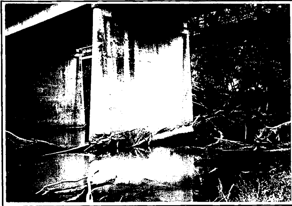
PIER NO. 3 (LOOKING FORWARD ON SURVEY)
