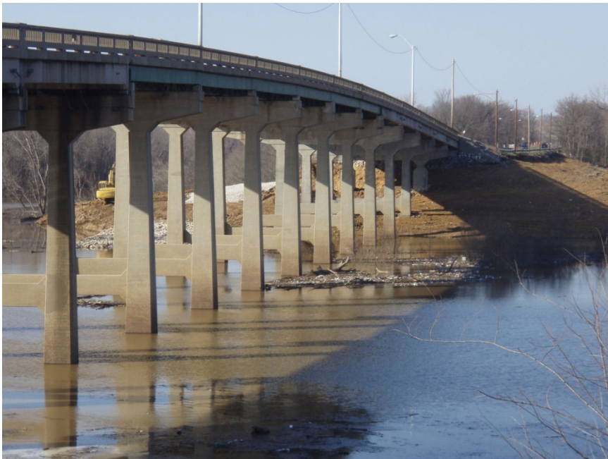
Figure 28. TN 003 (US Rt. 51) over the Wolf River, Shelby Co., TN.
