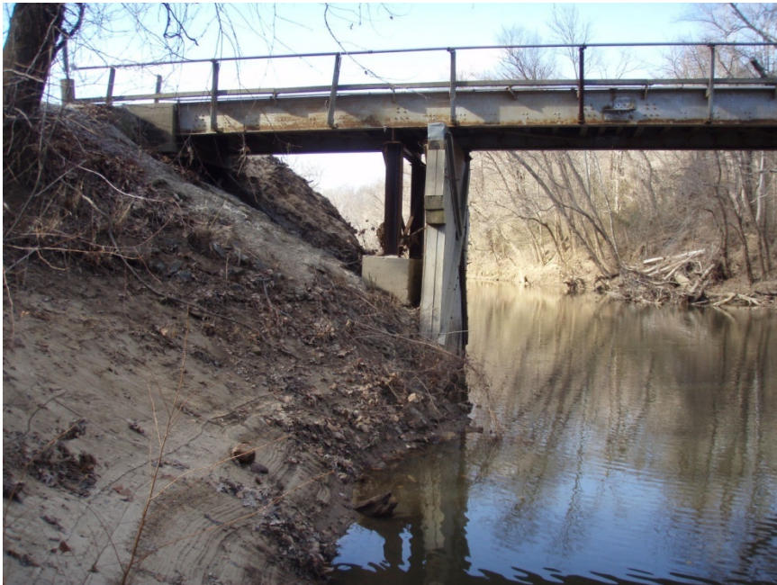
Figure 22. VA 621 bridge over the Mehrrin River, Lunenburg/Mecklenburg Co. line, VA.
