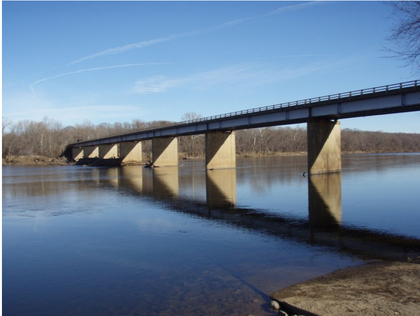
Figure23. VA 522 bridge over the James River, Goochland/Powhatan Co. line, VA.
