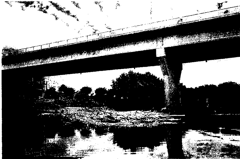
6. Pier 3, upstream nose. Note the large build-up of timber debris.
