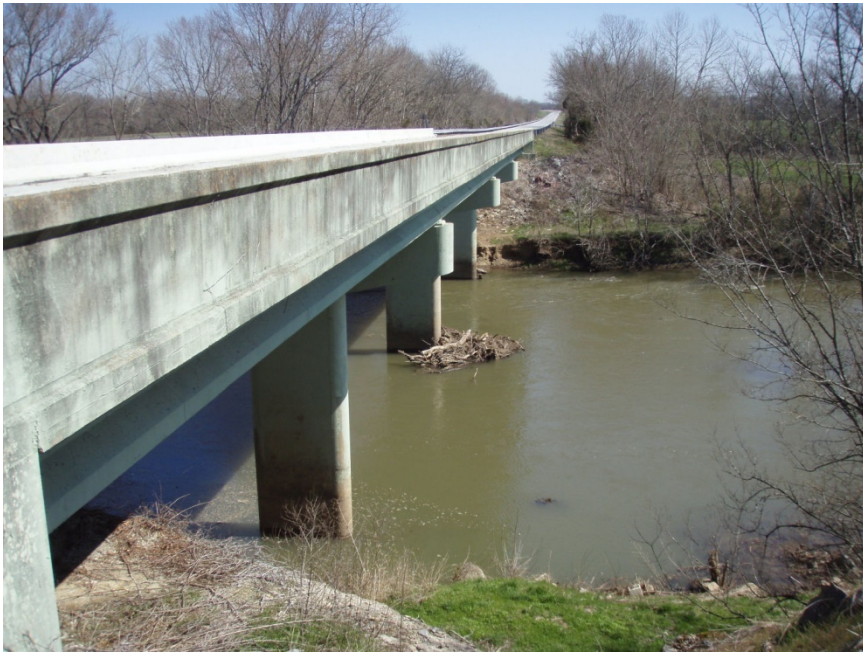
Figure 30. TN 274 over the Elk River, Lincoln Co., TN.
