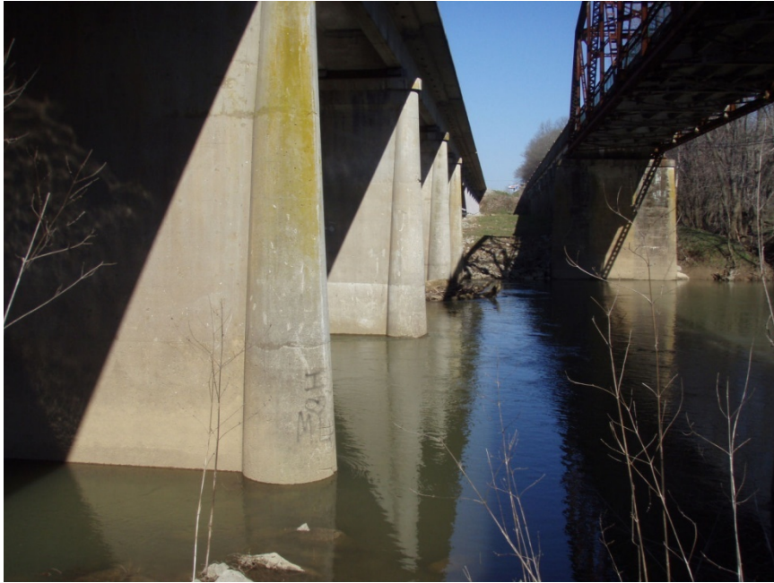
Figure 29. TN 007 (US Rt. 31) over the Elk River, Giles Co., TN.
