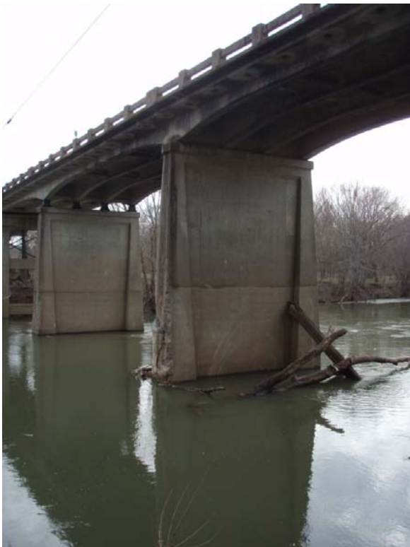
Figure 26. TN 250 bridge over the Harpeth River, Cheatham Co., TN.
