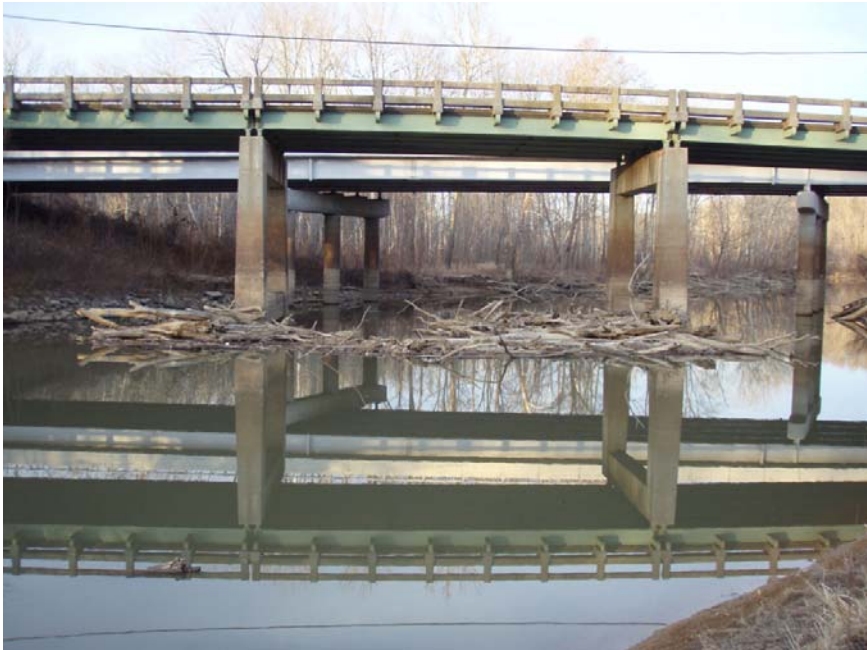
Figure 16. US Rt. 58 bridge over the Hycro River, Halifax Co., VA.
