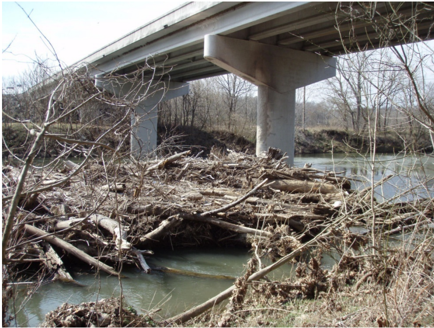
Figure 25. TN 249 bridge over the Harpeth River, Cheatham Co., TN.
