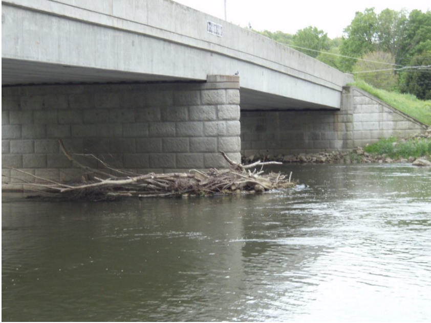
Figure 11. PA 3017 over French Creek, Venango County, northwest of Franklin, PA.
