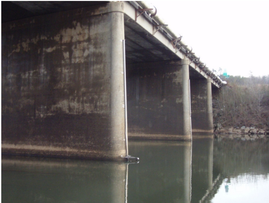
Figure 19. VA 668 bridge over the Staunton River, Pittsylvania-Campbell Co. line, VA.
