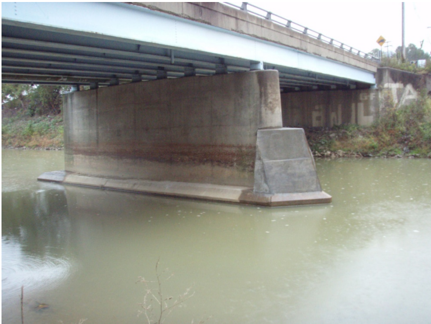
Figure 34. PA 3031 over Chartiers Creek, Allegheny County, PA.
