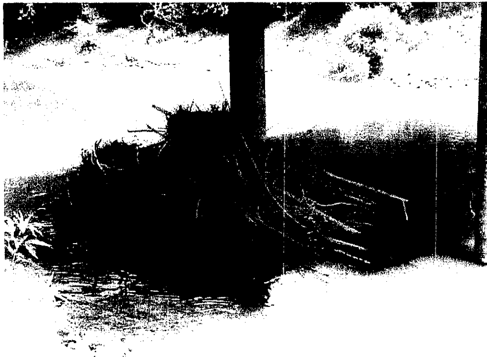
Photo No. 10 – Bent No. 29 (Debris at Upstream Column – 7/25/00)
