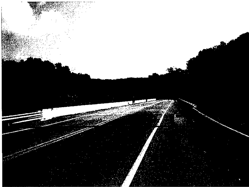
VIEW ACROSS TOP OF DECK
