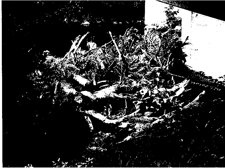
HEAVY DRIFT AT PIER #3
