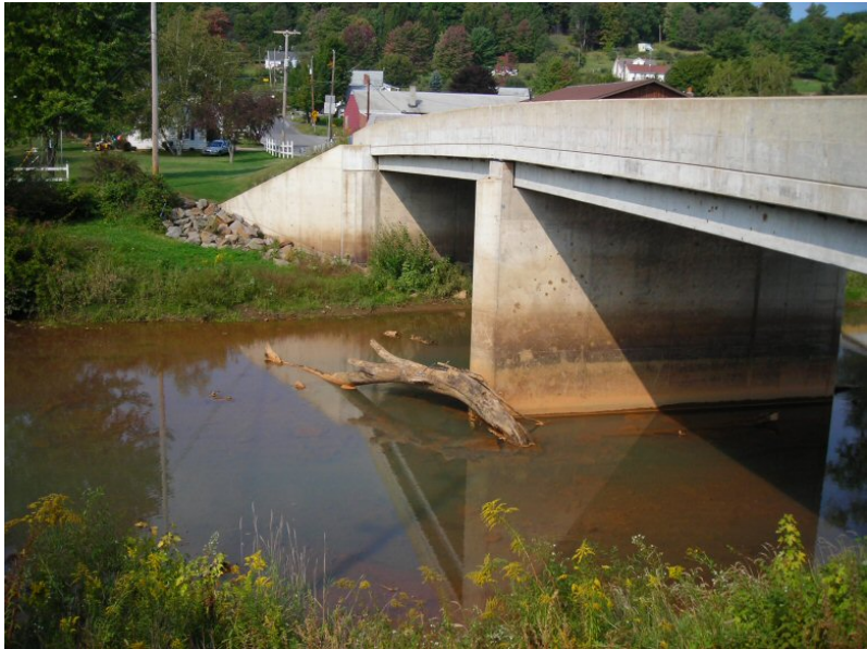
Figure 8. PA 3019 over Clearfield Creek, Clearfield County, Coalport, PA.
