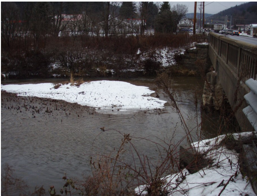
Figure 10. PA 153 over Bennett Branch, Clearfield County, near Penfield, PA.
