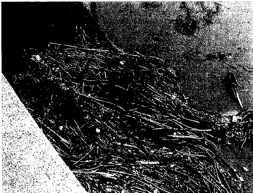
VIEW OF CHANNEL LOOKING RIGHT AT DRIFT
