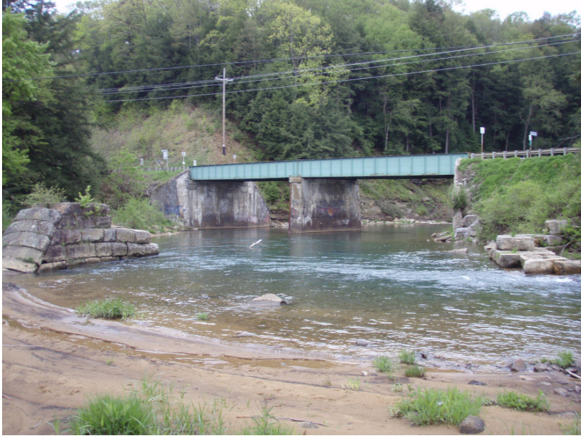
Figure 13. PA 2013 bridge over East Sandy Creek, Venango County, PA.
