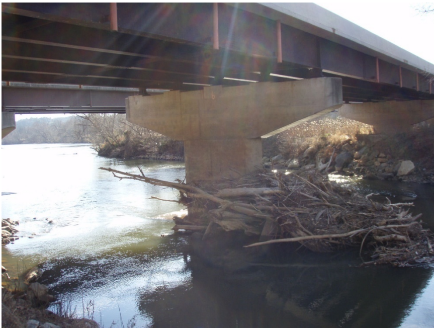
Figure 18. US Rt. 29 bridge over the Dan River, Pittsylvania Co., VA.
