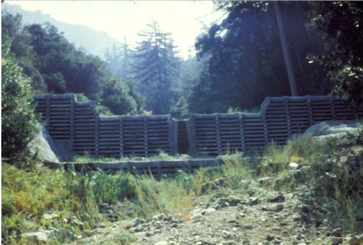
Figure 3. In-channel debris basin (from Bradley et al. 2005).
