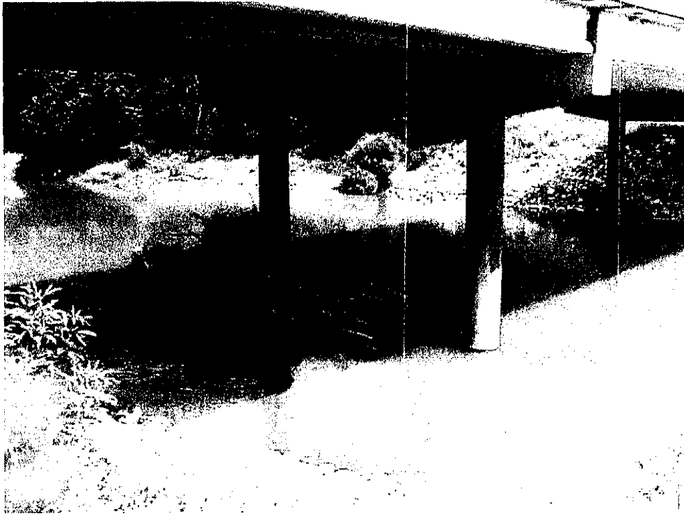
Photo No. 9 – Bent No. 29 (Back – 7/25/00)
