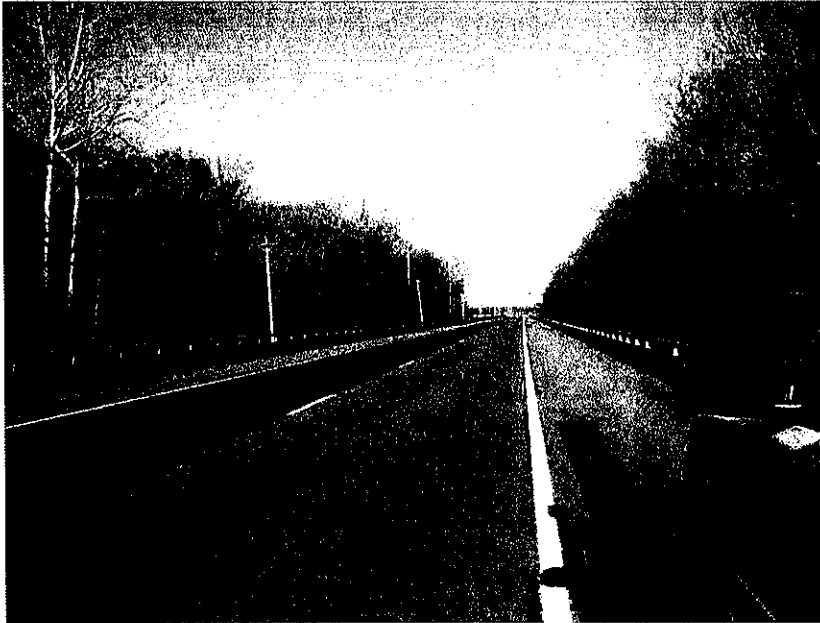
VIEW ACROSS TOP OF DECK
