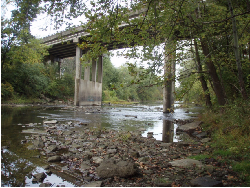
Figure 33. PA 588 over Connoquenessing Creek, Beaver County, PA.
