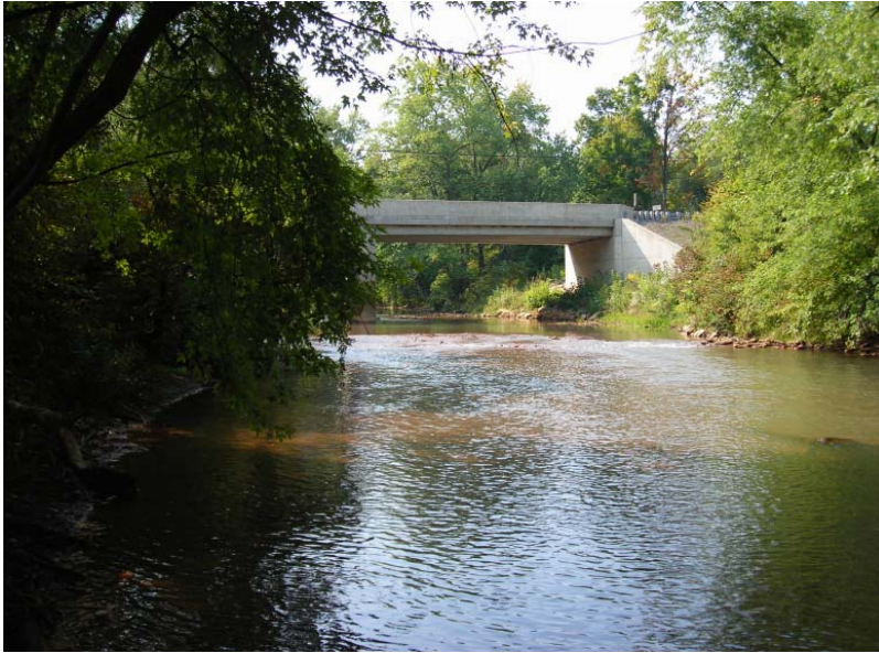
Figure 7. SR 3012 bridge over Clearfield Creek, Clearfield Co., Coalport, PA.
