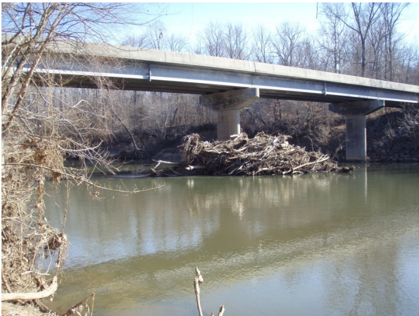
Figure 20. VA 880 bridge over the Dan River, Pittsylvania Co., VA.
