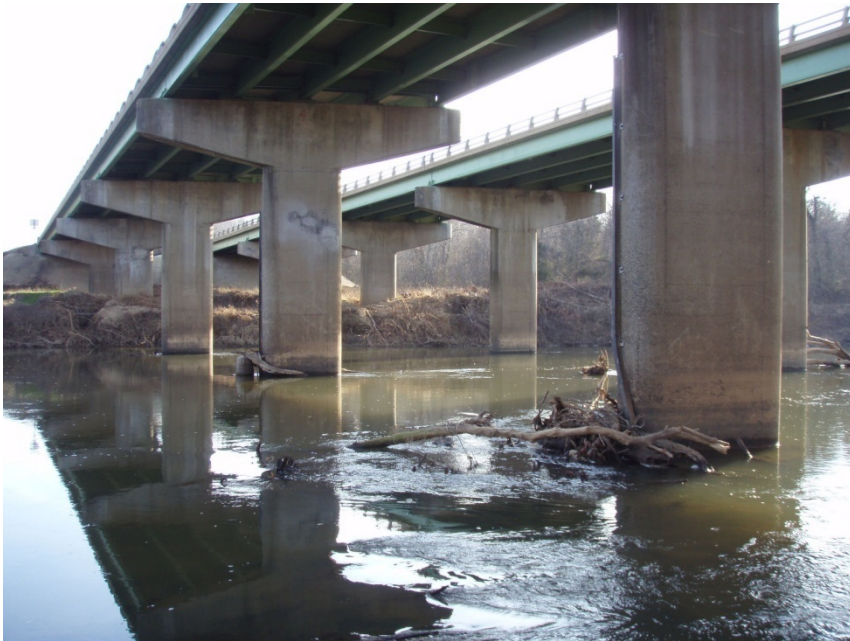
Figure 14. US Rt. 360 bridge over the Staunton River, Charlotte-Halifax Co. line, VA.
