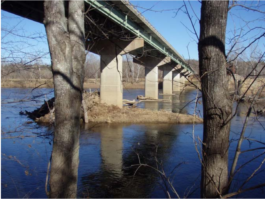
Figure 15. VA 45 bridge over the James River, Cumberland-Goochland Co. line, VA.
