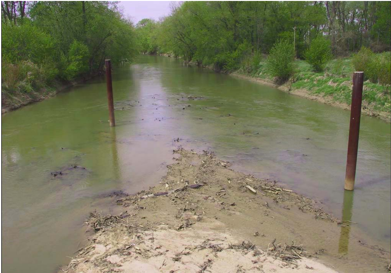
Figure 5. Cylindrical pile debris deflectors installed in an Indiana River (from Bradley et al. 2005).
