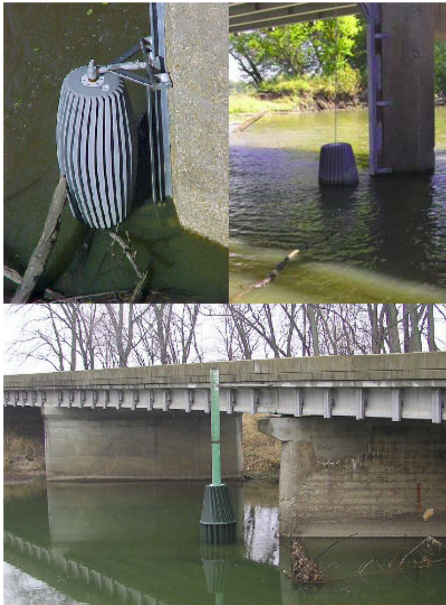
Figure 6. Clockwise from upper left, debris sweepers installed using the first-, second-, and third-generation pier attachment systems (from Debris Free, Inc.).
