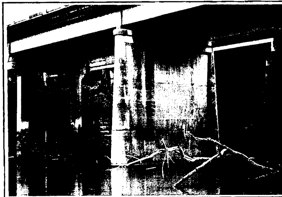
PIER NO. 4 (LOOKING FORWARD ON SURVEY)
