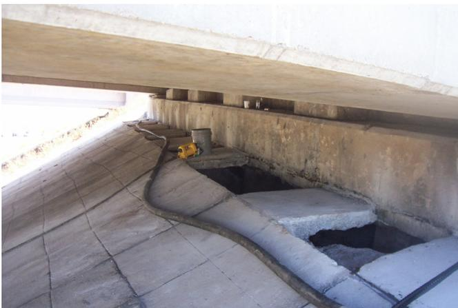
Scheduled routine inspections on this bridge revealed a void beneath the concrete slope protection.
