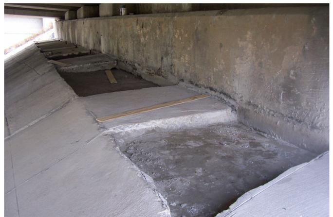
The void was filled with flowable fill to avoid damage to the bridge.
