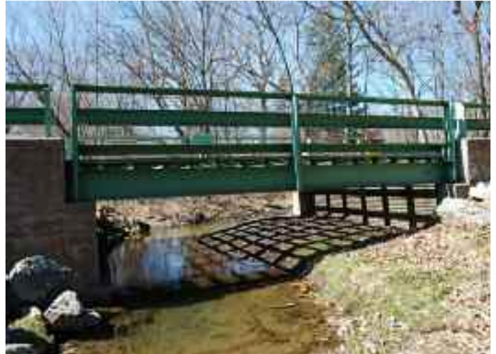
Northampton County will replace 28 bridges and rehabilitate five structures using P3 project delivery.
