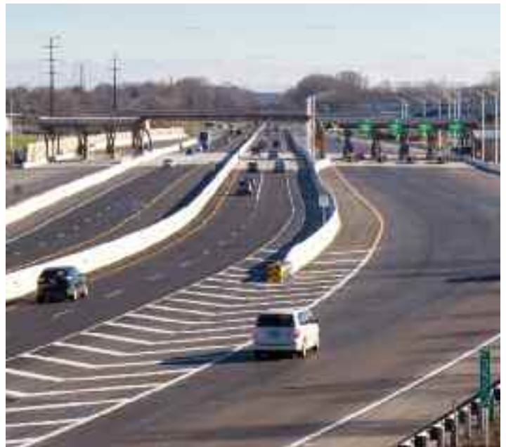
The selected private entity will install fiber optic cable and a wireless network throughout the PTC's 550-mile corridor.
