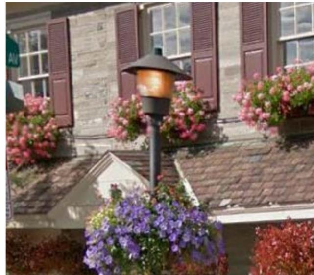
Light fixture heads are in very poor shape with opaque yellow lenses and damage. Lens conditions impact efficiency and cause more glare problems.
