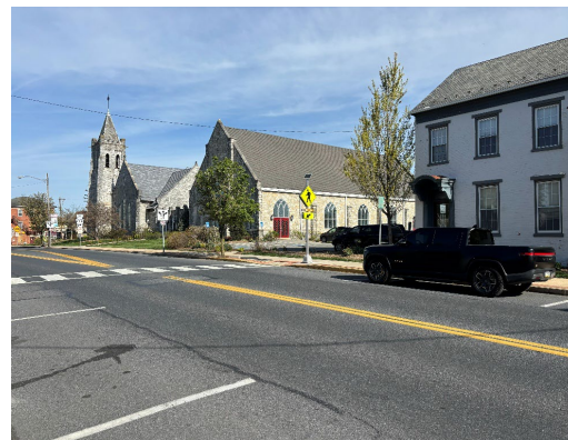
Figure 2: Pedestrian safety improvements are eligible for ARLE funding Photo: PennDOT Municipal Resources
