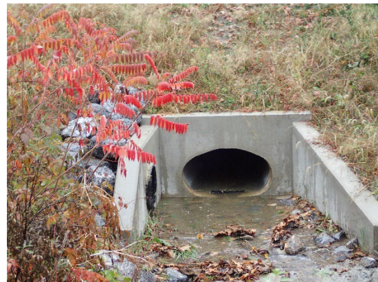
This is a newly placed stormwater pipe culvert near Washington Avenue in Logan Township. Photo: PennDOT
