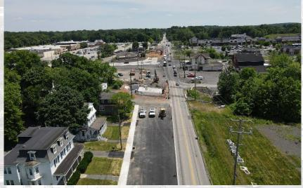
The contractor is currently constructing the top-slab of the culvert, which will be followed by construction of the concrete approach slabs.
