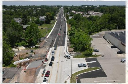
Excavation for the second stage of the precast box culvert near Kohls has been completed for the southern portion, and the phased construction of the new twin-cell culvert will take place this summer. After the completion of the culvert, the concrete pavement will be constructed towards the SR73 intersection.
