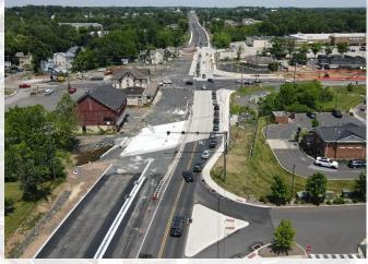
The contractor has also constructed the cast-in-place wing walls and the concrete approach slabs for the second stage of the box culvert near CVS. Final roadway paving and placement of pavement markings will take place this summer, between Swede Road and Wawa.
