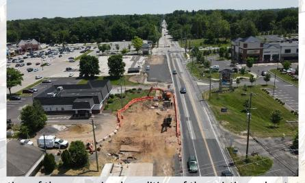
Following the relocation of the gas main, demolition of the existing culvert near Wells Fargo will begin this summer, after which the contractor will begin the installation of the new concrete box culvert.
