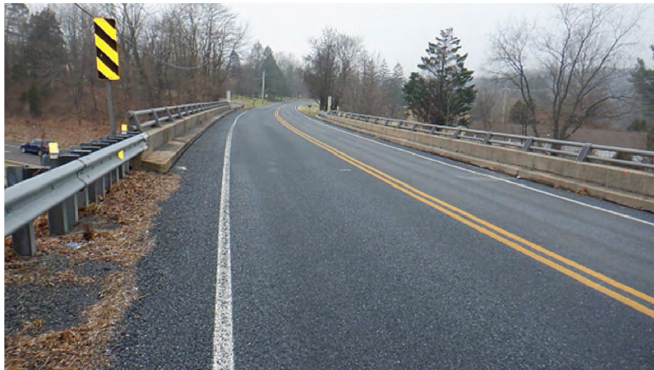
SR 3024 - LOOKING WEST
