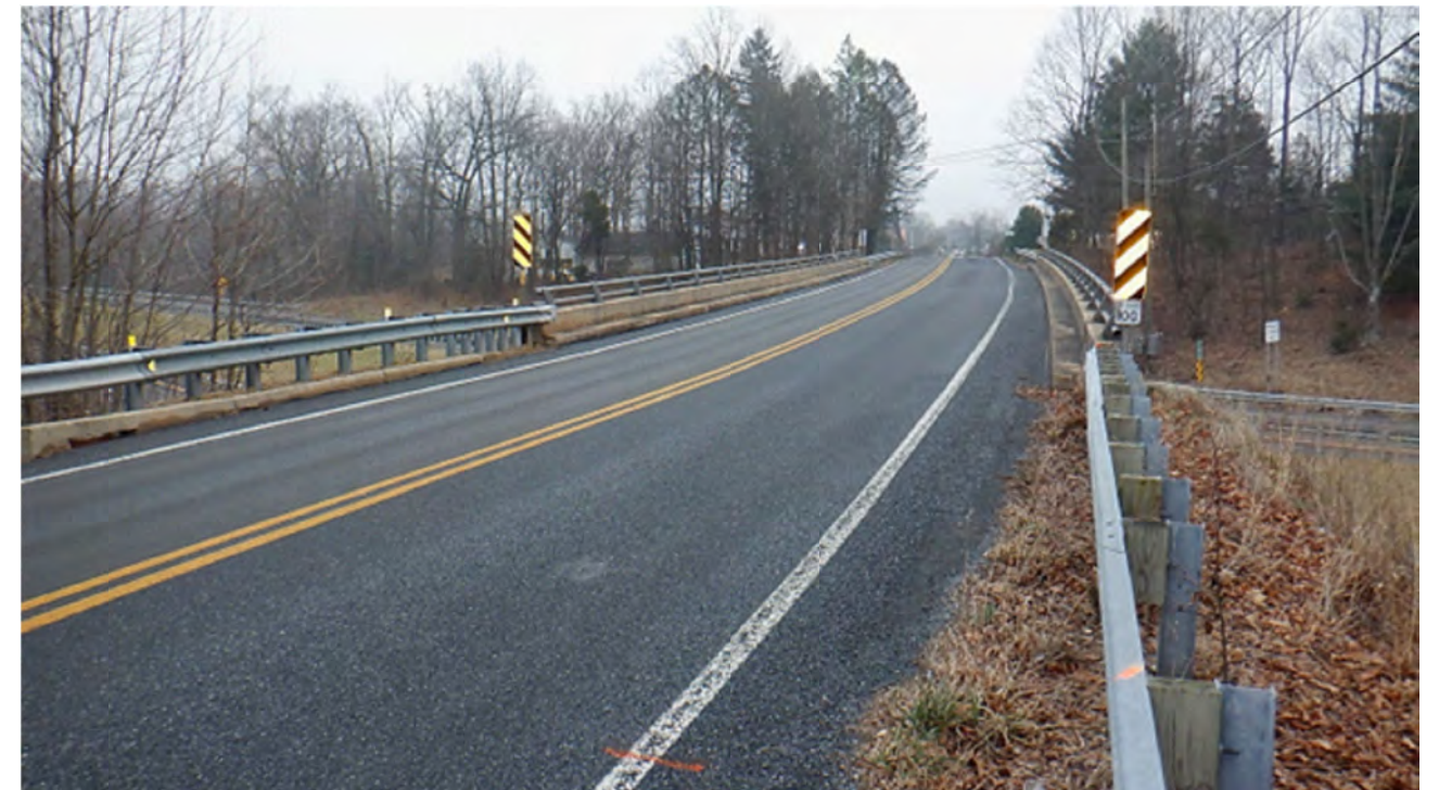
SR 3024 - LOOKING EAST
