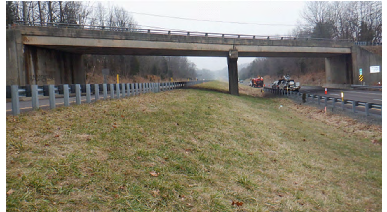
SR 3024 BRIDGE OVER I-176 - LOOKING SOUTH
