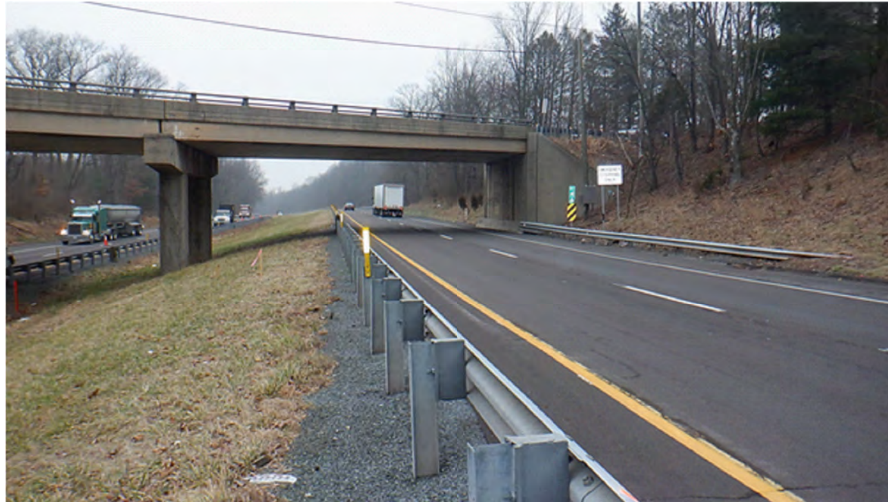
SR 3024 BRIDGE OVER I-176 - LOOKING NORTH
