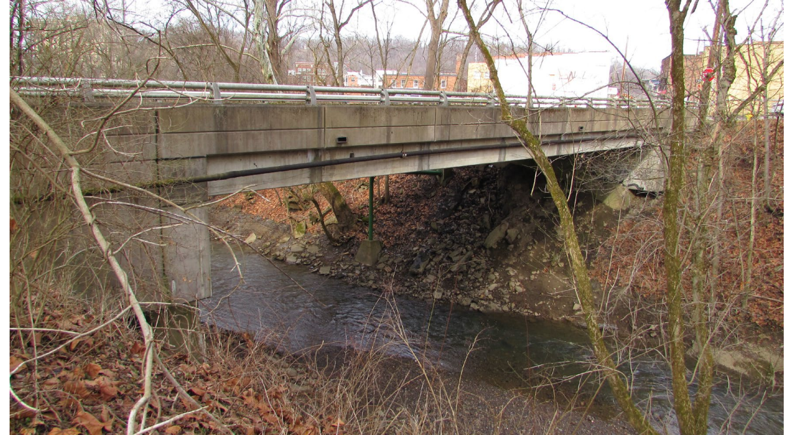
Upstream Elevation View of Bridge
