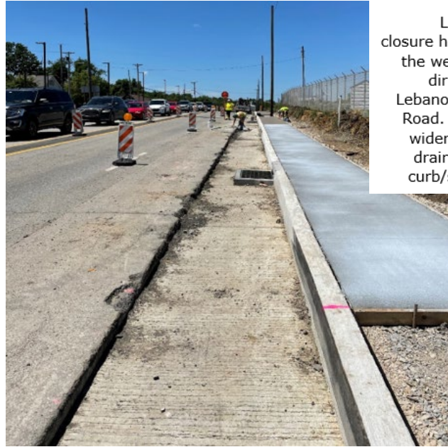
New mountable curb/pavement islands. Both east and west bound lanes have newly placed binder. Wearing course will be placed later in the year.
