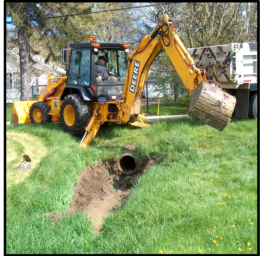
Drainage outlet blocked by private property owner Department permitted to open under the Ditch and Drainage Act
