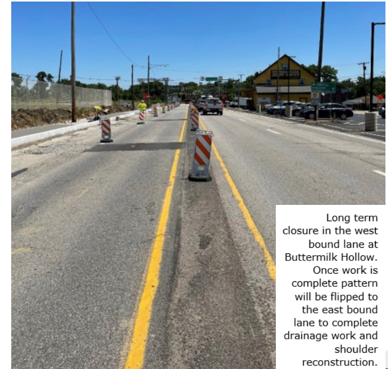
New mountable curb/pavement islands. Both east and west bound lanes have newly placed binder. Wearing course will be placed later in the year.
