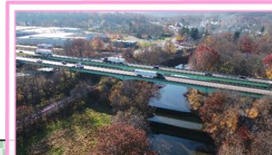
I-79 over PA 68 and Connoquenessing
