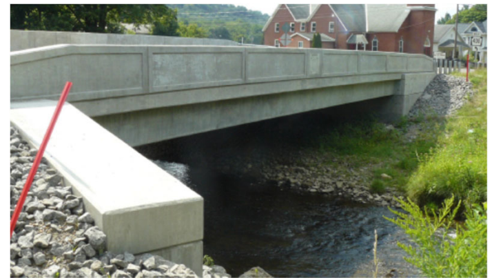
Above: Panel design will be very low maintenance and easy to repair in the future.
