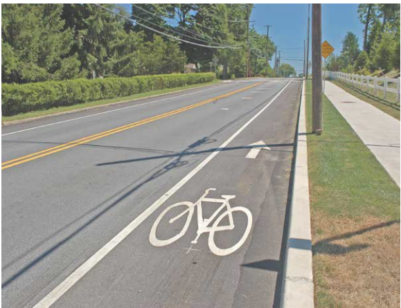
Dimensions 5 – 7 feet wide (4 feet minimum, exclusive of gutter)
