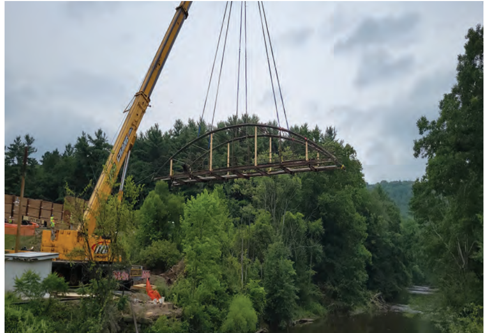
Messerall Road Bridge in Crawford County during relocation
