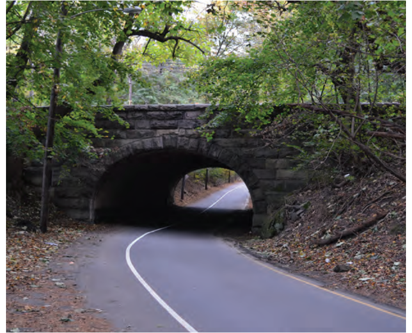
Elliptical Arch, Belmont Avenue Bridge in Philadelphia
