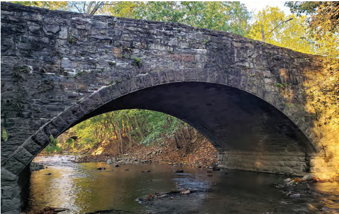
Circular Arch, Bridge in Newport Borough, Perry County
