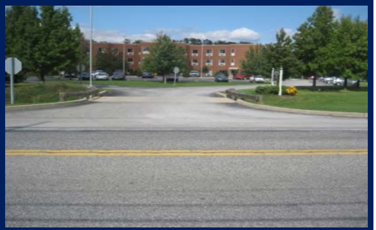
Figure 1.1.2- Culvert conveys water under driveway.
