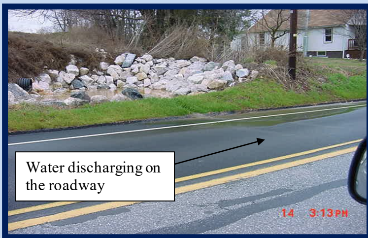
Figure 1.2.3- A photo of storm water that is not adequately retained and overflow water ponds on the roadway surface.
