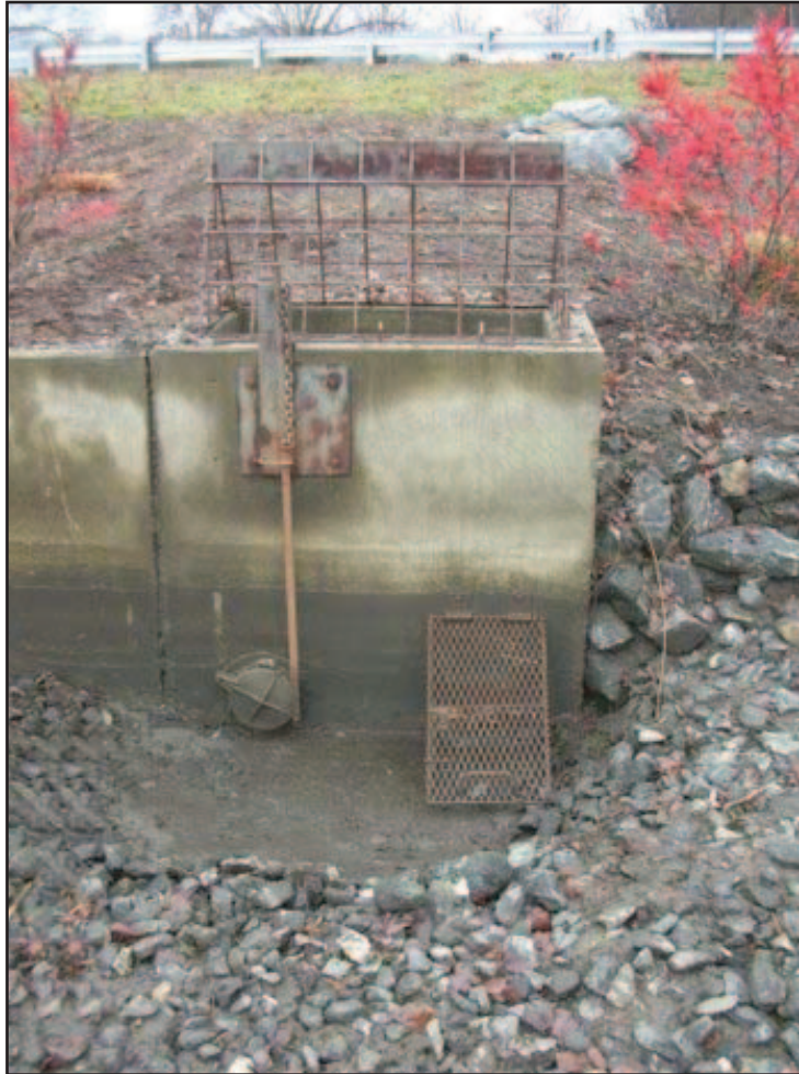
Figure 5.2.3: Lift-Type Sluice Gate (c/o NCDot-HSP-2010-01)
