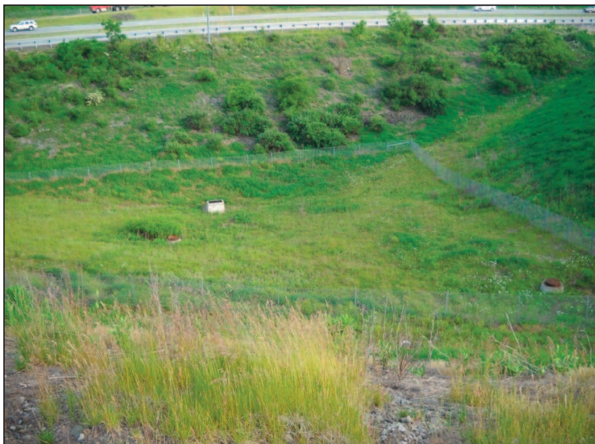
Figure 5.1.1: Dry Extended Detention Basin
