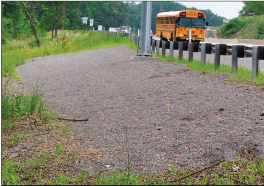
Figure 5.10.1: Media Filter Drain with Unvegetated Surface
