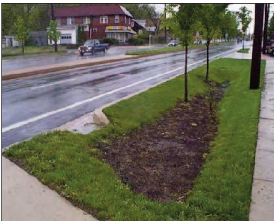
Figure 6.3.1: Inflow System- Curb Cut
