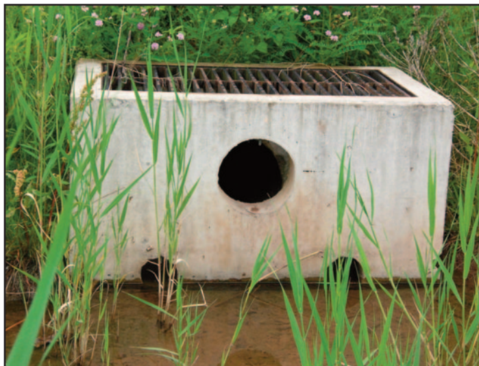
Circular orifices without trash rack
