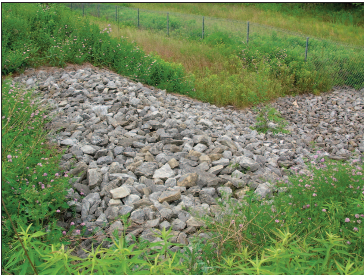
Figure 6.9.1: Earthen Emergency Spillway
