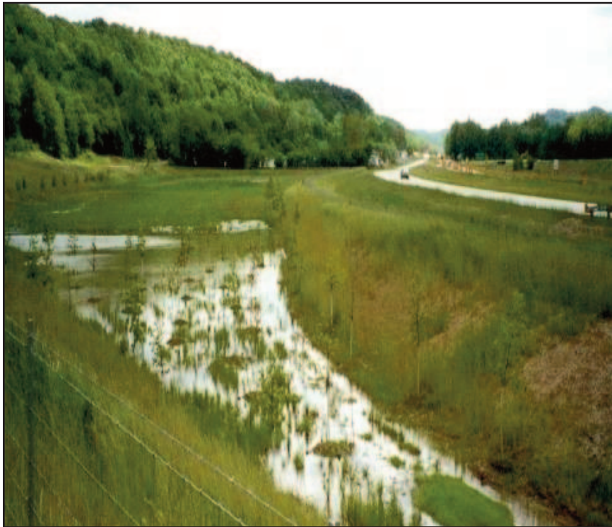
Figure 5.7.1: Stormwater Wetland – Extended Detention Shallow Wetland
