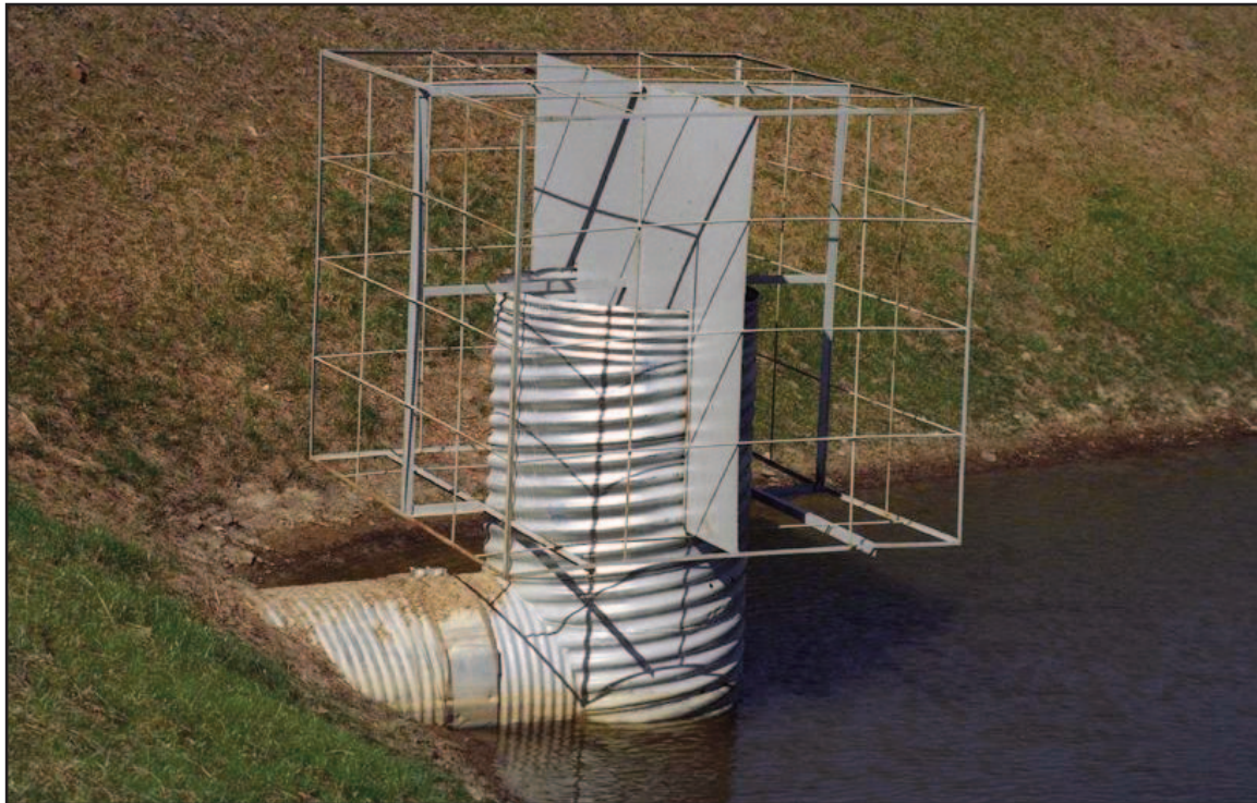
Metal Riser with Trash Rack and Vortex Plate (photo c/o: PADEP E&S Manual)
