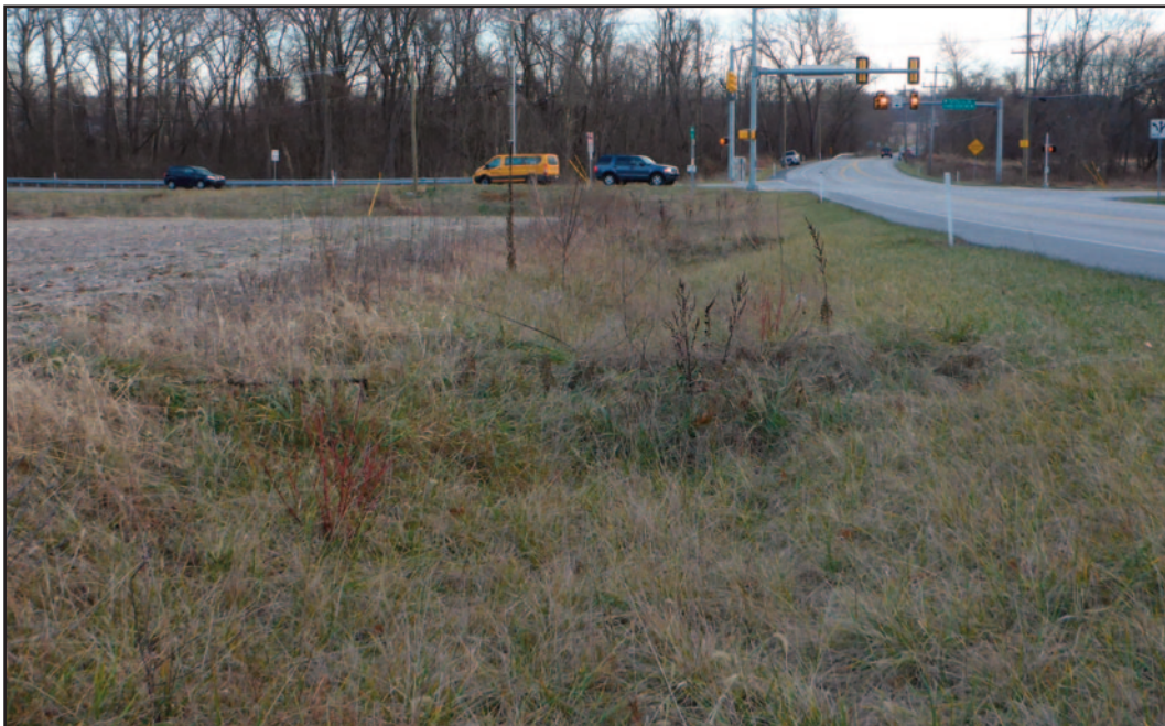
Figure 5.11.2: Vegetated Swale with Check Dams (VSC)
