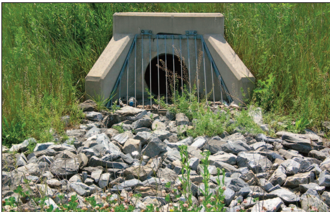
Headwall with Trash Rack Figure 6.8.1: Structures and Appurtenances
