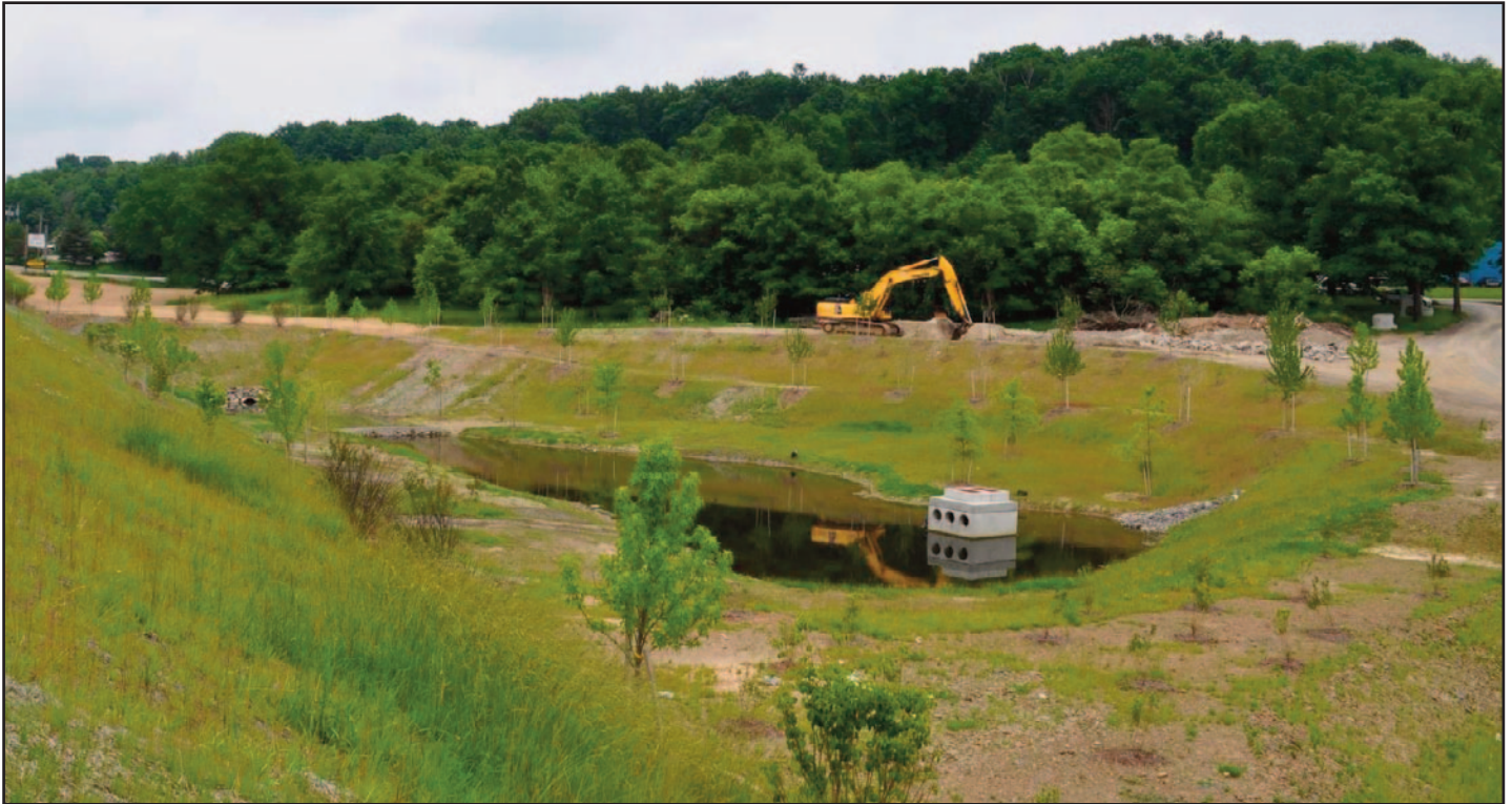
Figure 5.2.1: Newly Constructed Wet Detention Basin
