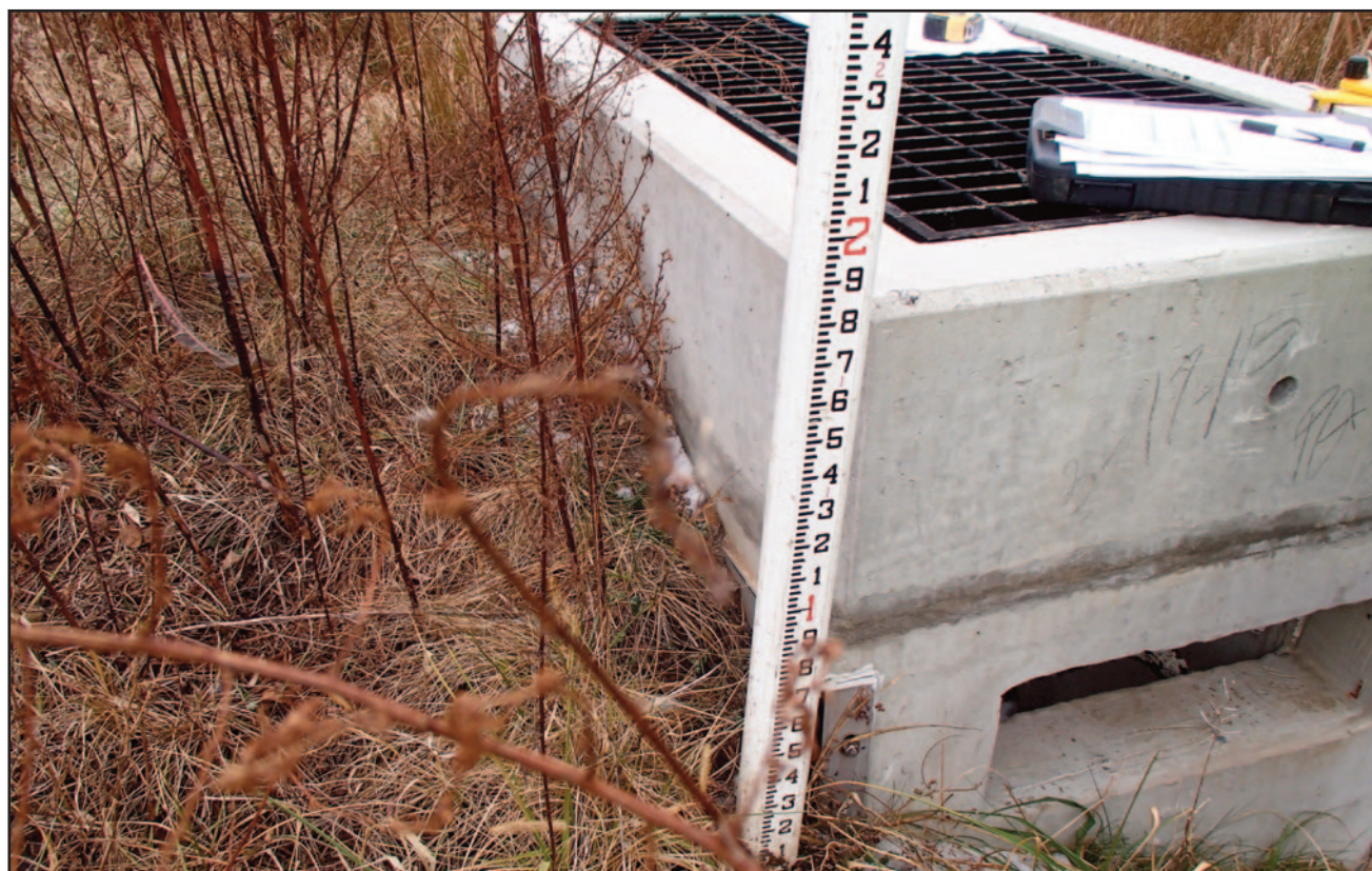
Figure 3.1.1 SCM Inspection in Progress
