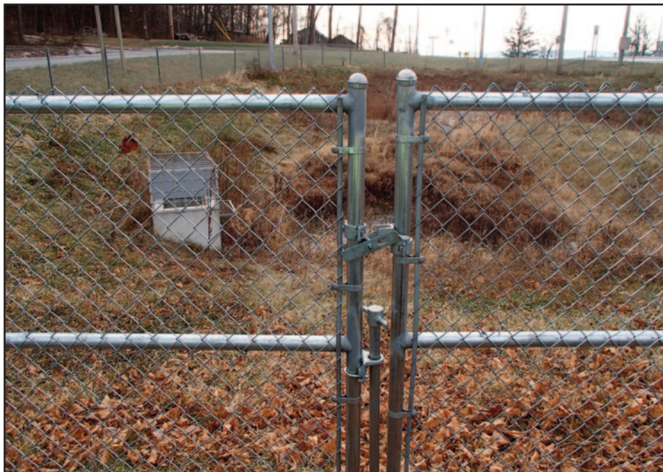
Figure 6.1.1: Fencing Surrounding an SCM
