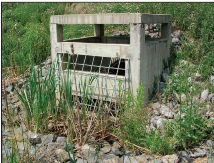
Rectangular weirs with side mounted trash rack
