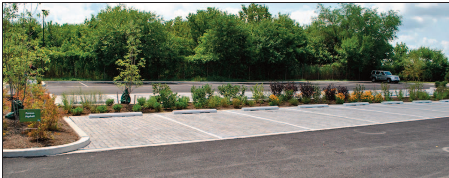
Figure 5.15.1: Pervious Pavement Pavers (PPP)
