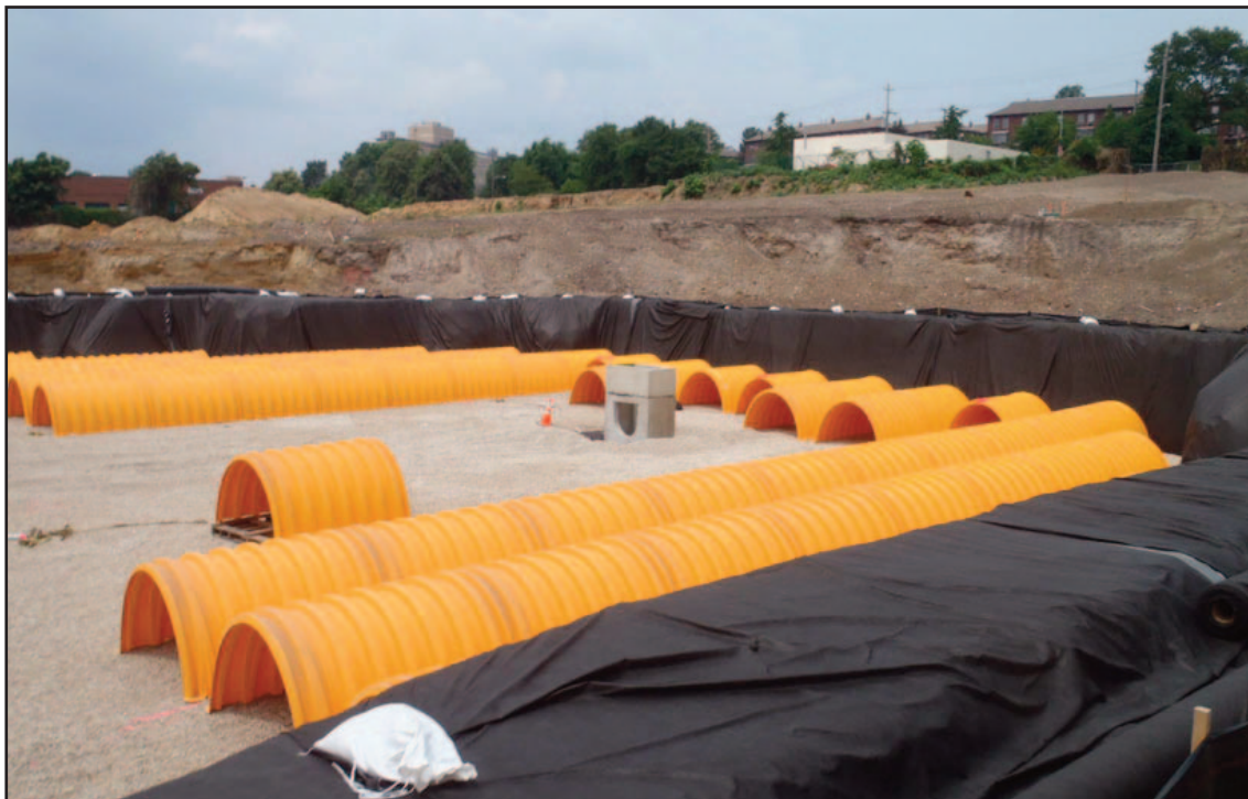
Figure 5.6.1: Subsurface Detention Storage Under Construction (photo c/o The Philadelphia Water Department, Stormwater Management Guidance Manual)
