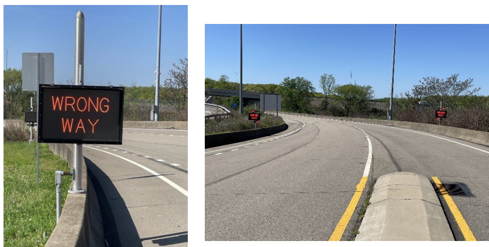
Figure 5.7.16–5: Example of LED-Enhanced Wrong-Way Signage
