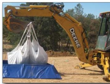
Figure 12. Extracting the concrete solids or gelled washwater
