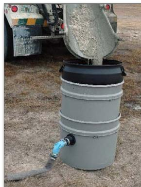
**Figure 3. Concrete washout filter**
