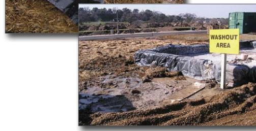
Figure 10. Leaking washout pit that has not been well maintained
