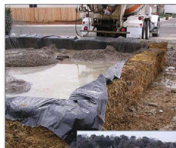
Figure 9. Hay bale and plastic washout pit
