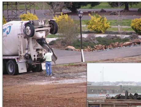
Figure 1. Chute washwater being dumped on the ground
