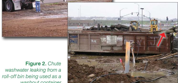
Figure 2. Chute washwater leaking from a roll-off bin being used as a washout container
