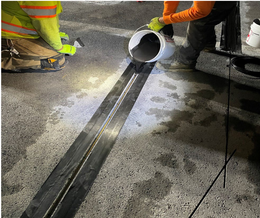
Installation of CAVC 833 on I-81 in Cumberland County
