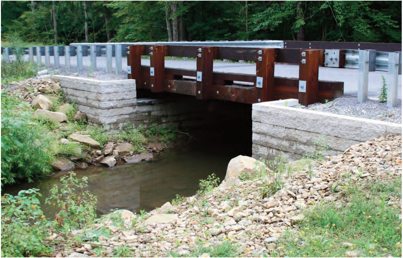
FIGURE 2. The 18-ft span Mount Pleasant Road Bridge constructed in Huston Township, Clearfield County, PA, in 2011.
