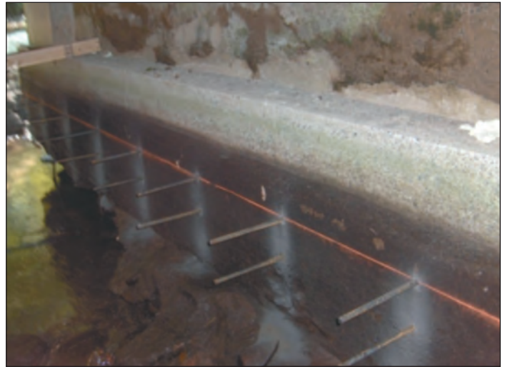
Installation of steel dowels, Concrete Forms, and Placement of new Concrete.
