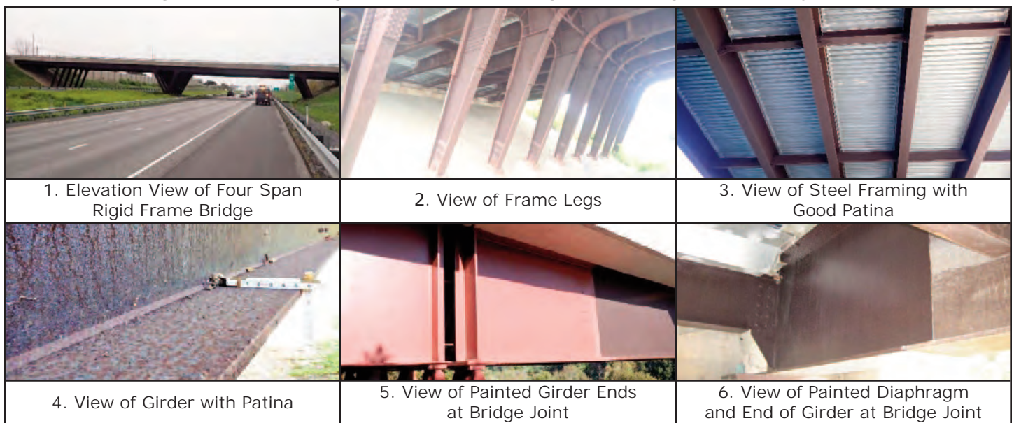
Figure 4-2 - Photographs of Weathering Steel Bridges in Pennsylvania
