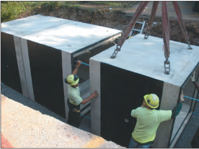
Consultant designed box culvert
