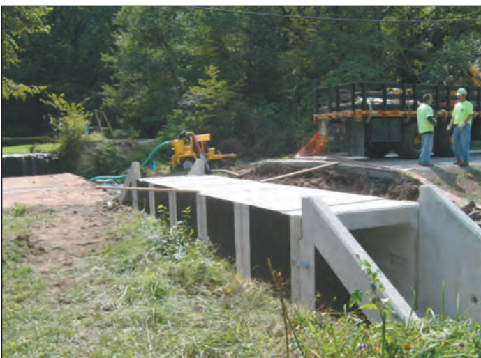
Backfill by Department Forces
