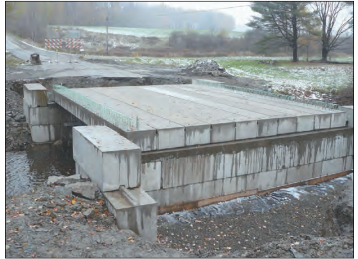
Installation of prestressed concrete channel beams by department forces.
