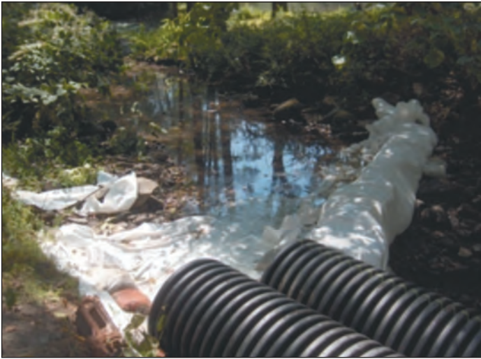
Diversion of stream flow utilized through HDPE Pipes. Installation of other E&S Control measures.
