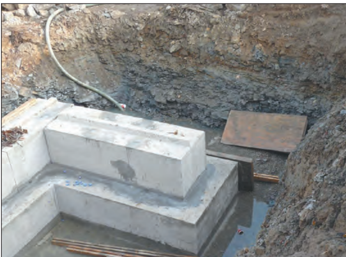
Installation of precast concrete block stem and wingwalls.
