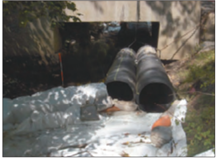
Diversion of stream flow utilized through HDPE Pipes. Installation of other E&S Control measures.
