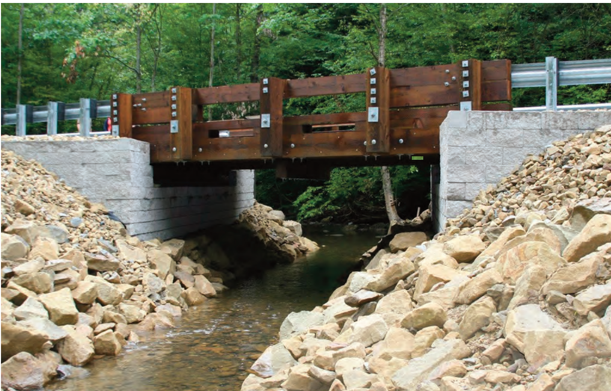
FIGURE 5. The Sandy Township, Clearfield County, Old Bliss Run Road Bridge over Mountain Run – Completed bridge.
