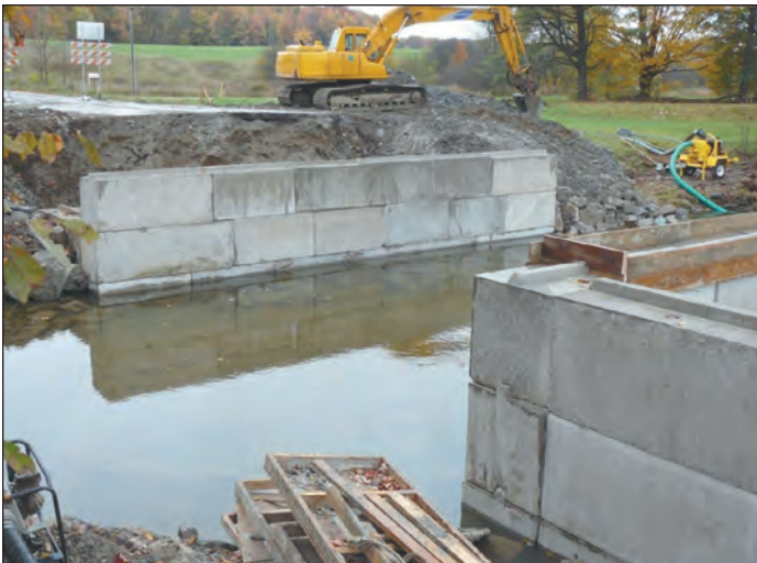
Installation of precast concrete block stem and wingwalls.
