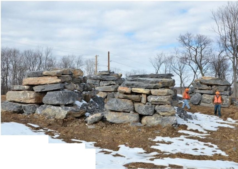
These examples of roost structures were clustered in the area with optimal solar exposure. These structures documented eastern small-footed bats using the structures months after construction was completed.
