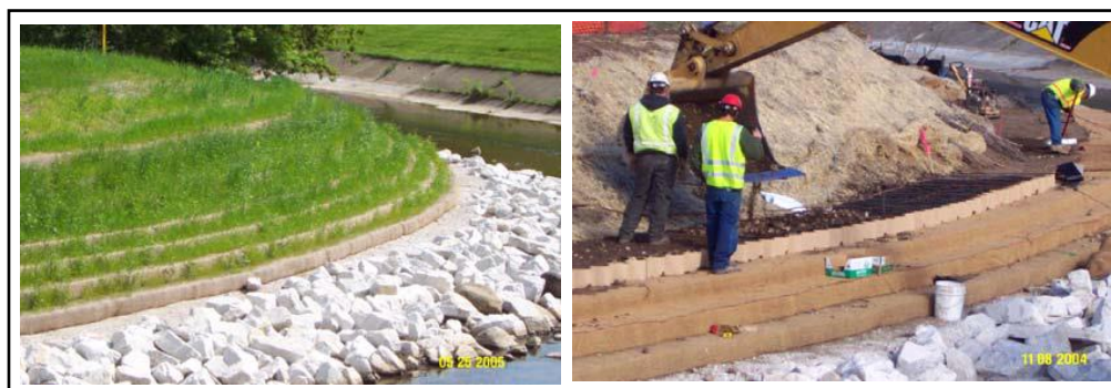
Figure 14.3.4-6 – Geocell for Erosion Control
