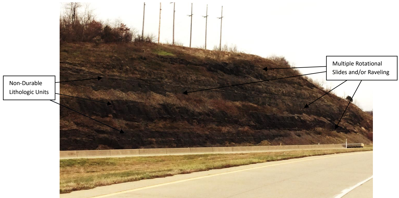
Figure 8.2-2 – Incompetent Design Section comprised of Non-Durable Lithologic Units
