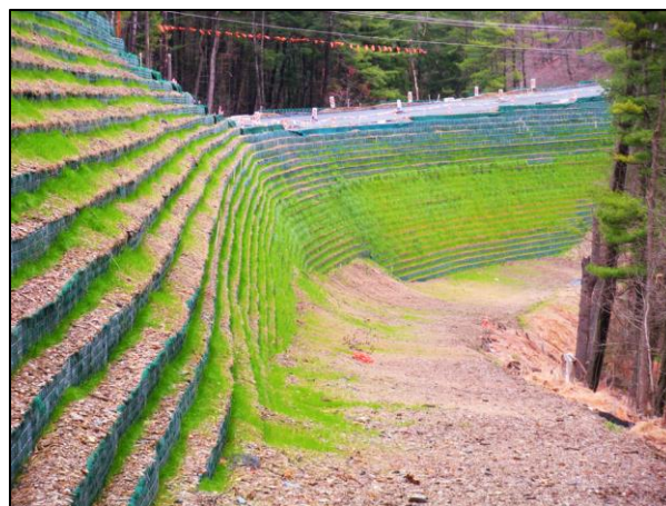
Figure 14.3.2.1-3 – Typical GRS Slope (0.5H:1V Slope; Height = 50 ft)
