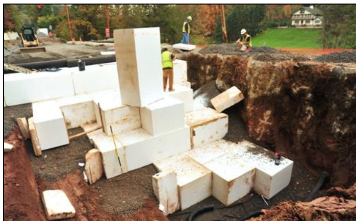
Figure 14.3.5-1 – EPS Geofoam Blocks (Typical Application – Lightweight Fill)
