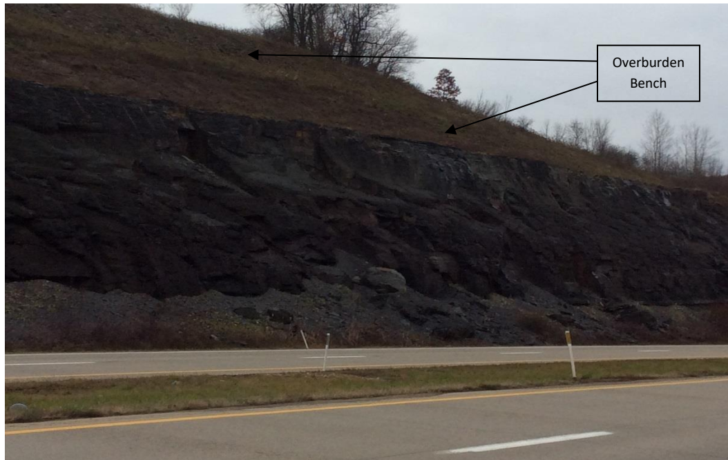
Figure 8.6.1-1 – Example of an Overburden Bench
