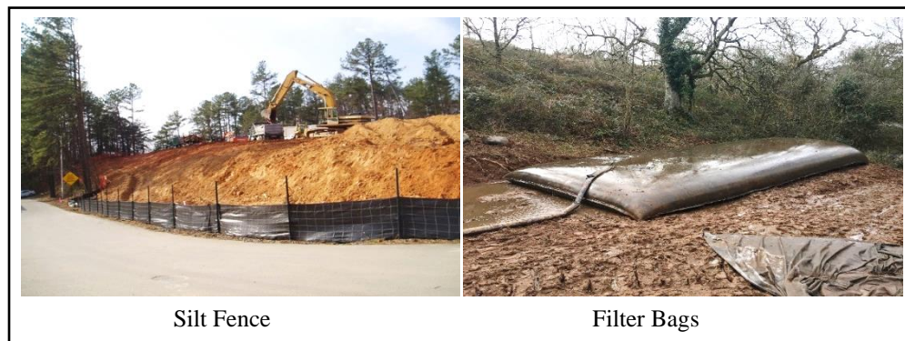
Figure 14.3.7.2-2 – Silt Fence and Filter Bags
