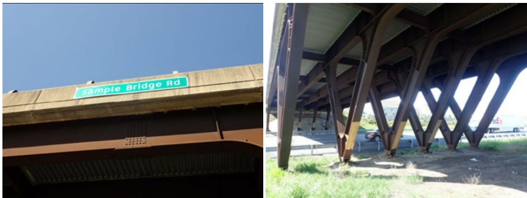
Figure 2 – UWS Delta K-Frame Bridge
