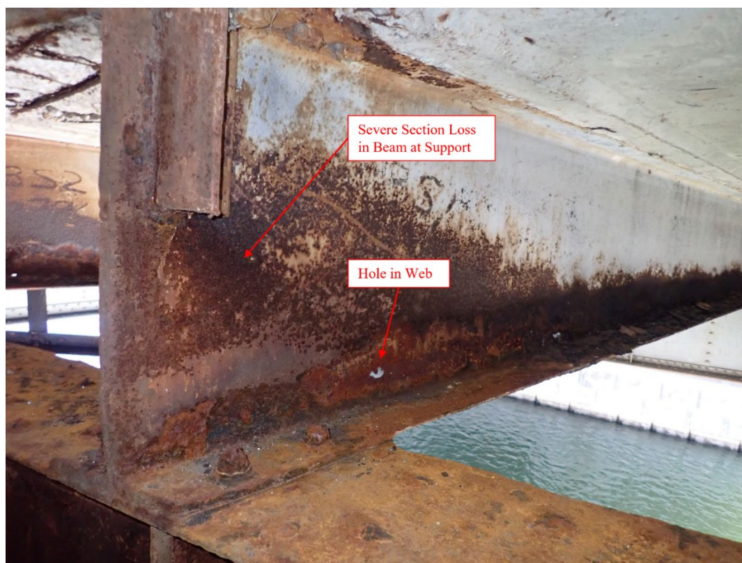
Figure 2.6.1.2-2 – Section Loss in Stringer Web at Support
