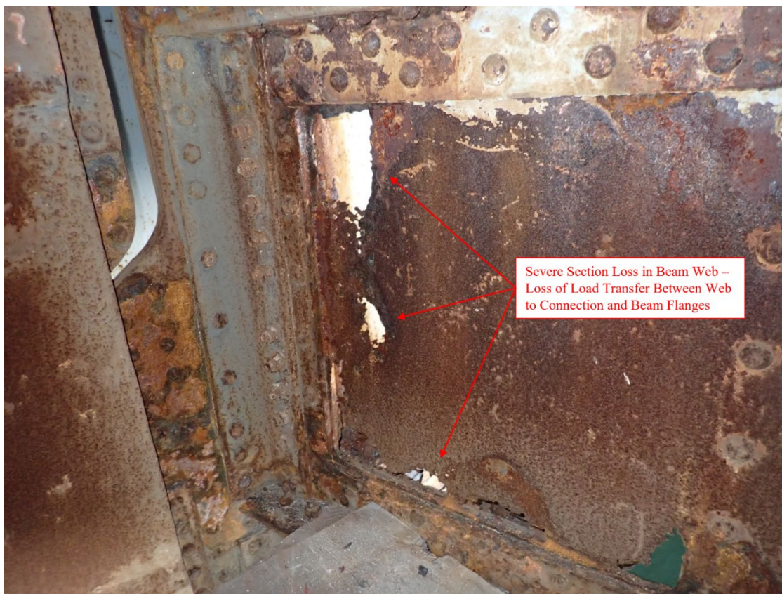
Figure 2.6.1.2-3 – Example of Severe Section Loss in Web Adjacent to Flange
