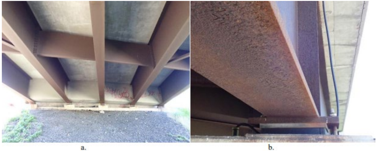
Figure 9 – Views of Patina Up Close and from a Distance Showing Different Results (Source: NSBA/AISC 2022)
