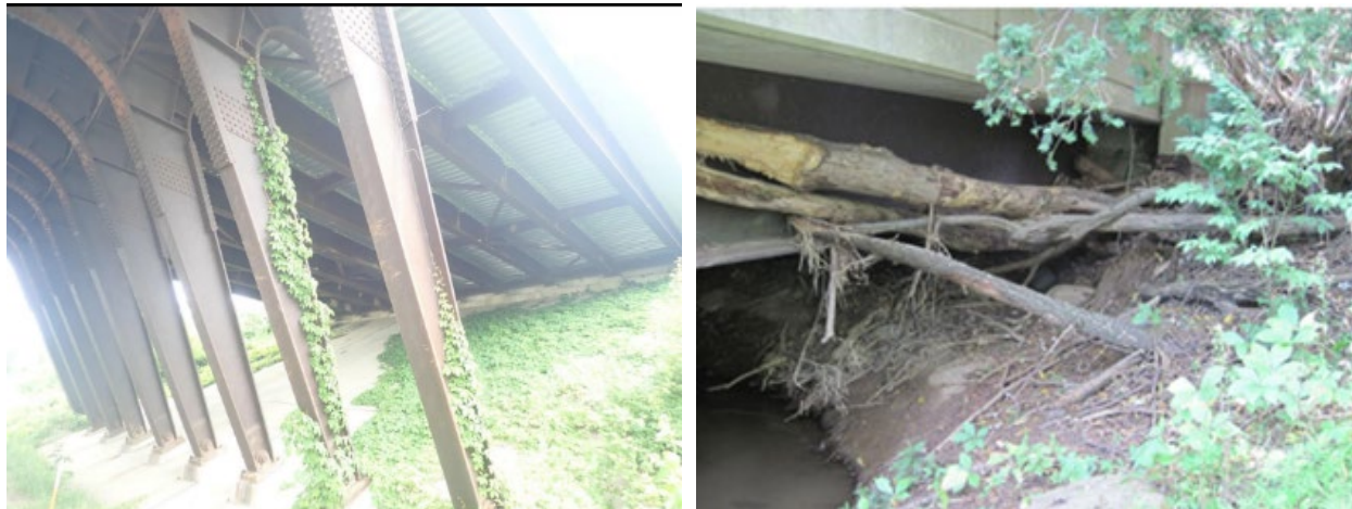
Figure 23 - Vegetative Growth and Waterway Debris Build-Up at UWS Bridges
