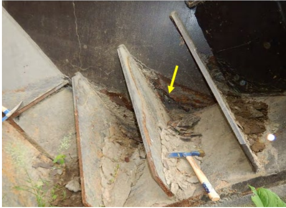
Debris Build-Up at Bottom of Frame Leg
