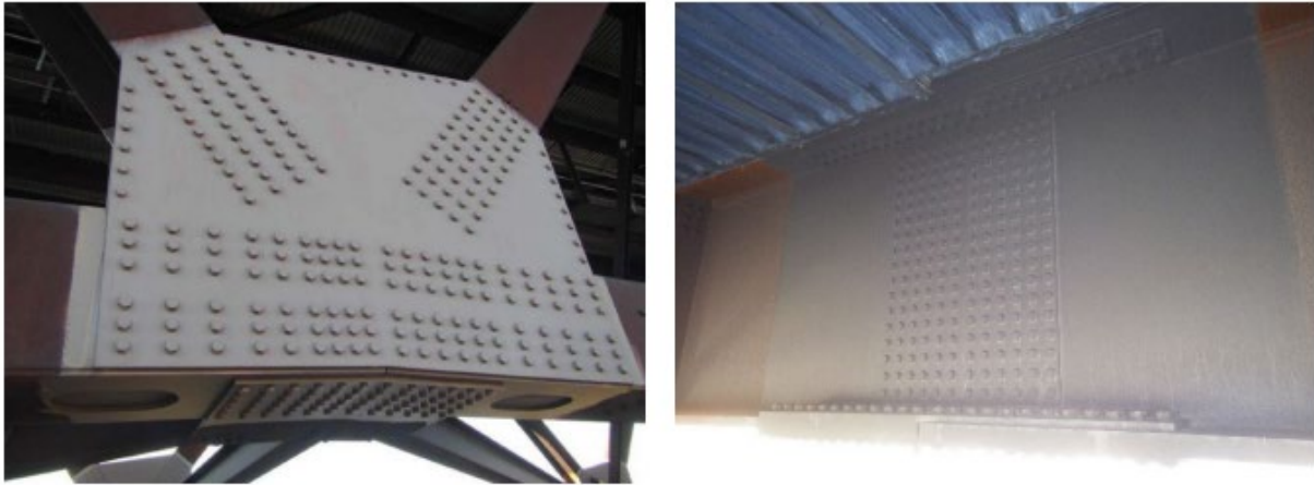
Figure 32 - Painted Gusset Plate and Girder Splice (Source: NSBA/AISC 2022)
