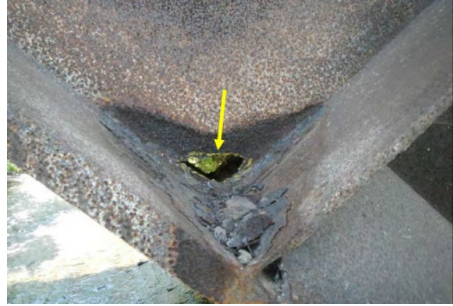
Debris Build-Up and Full Depth Web Corrosion at Frame Leg, Intersection of Flange/Web/Transverse Stiffener
