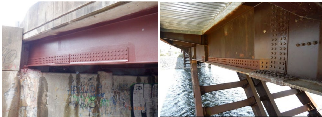
Figure 34 - Bolted Repair to Lower Section of UWS Girders
