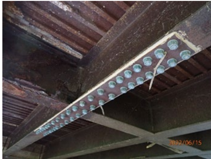
Figure 27 - View of Sealed Crevice at Bolted Cover Plate
