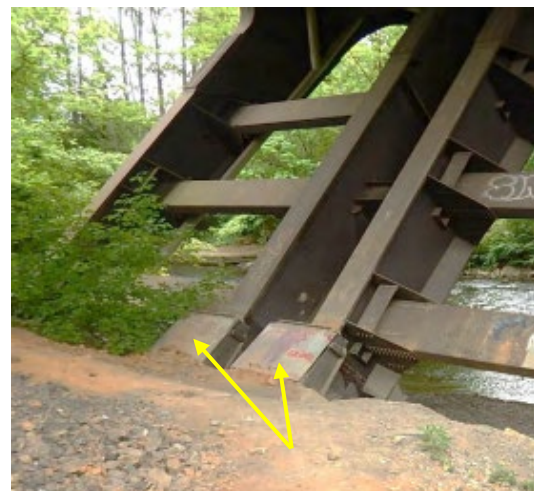
Figure 19 – Bearing Anchorage of UWS Frame Bridge: Views of Ineffective Asphalt Filling and Effective Watertight Steel Panel Retrofit
