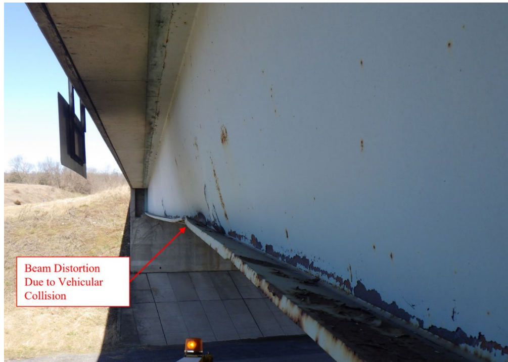
Figure 2.6.1.2-1 – Example of Beam Distorted Due to Vehicular Collision
