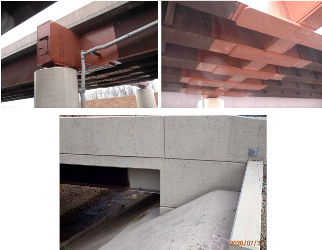
Figure 5 - Painted Steel Box Cross Girder, Painted End of Girder
