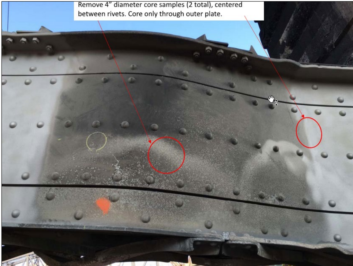
Figure 3 – Location of 4-inch diameter Cores
