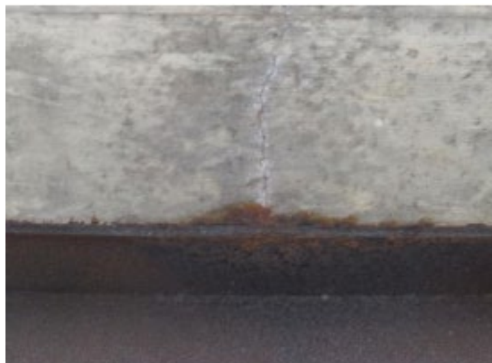
Figure 22 – Top Flange Deterioration Beneath Concrete Deck Crack (Source: Crampton et al., 2013)
