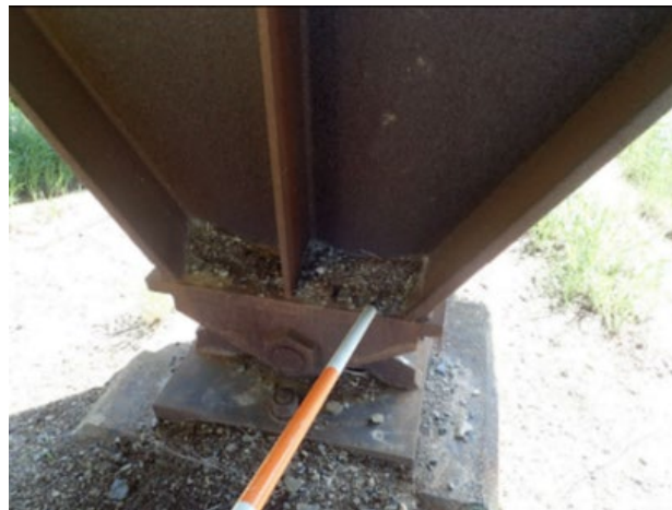
Debris Build-Up at Bottom of Frame Leg
