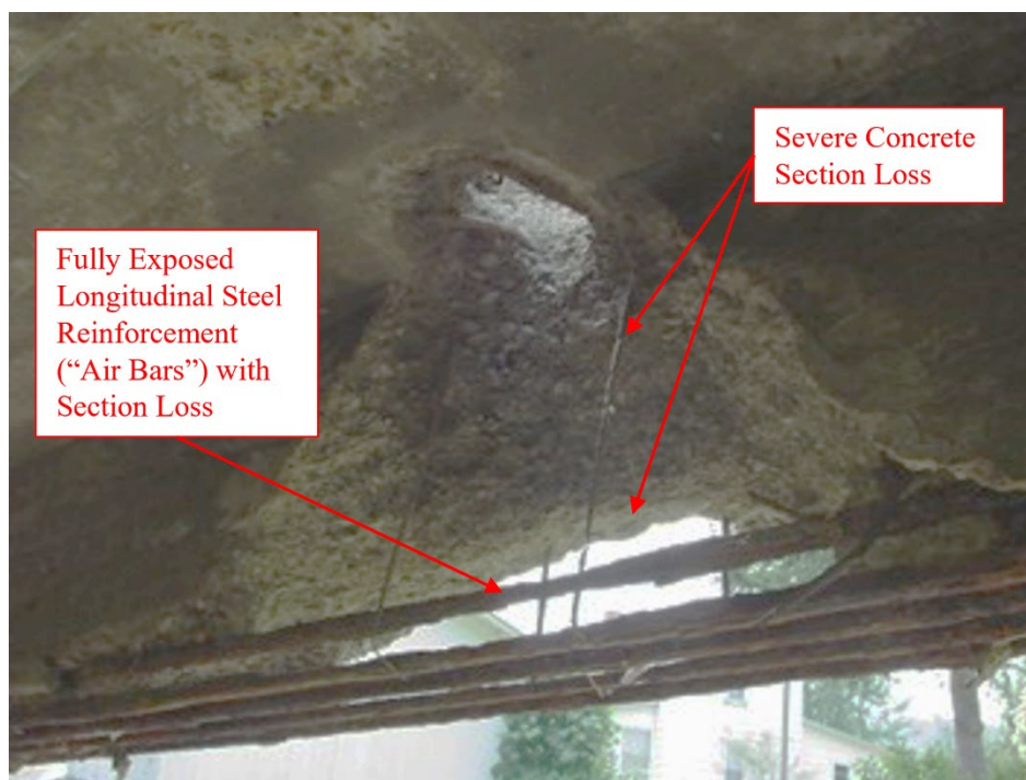
Figure 2.5.1.2-4 – Example of Ineffective Reinforced Concrete T-Beam – "Air Bars"
