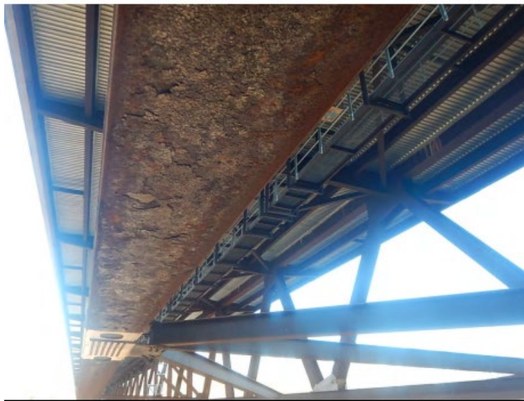
Figure 7 – Extensive Rust Laminations Along the Lower Chord of a Modern Deck Truss Bridge
