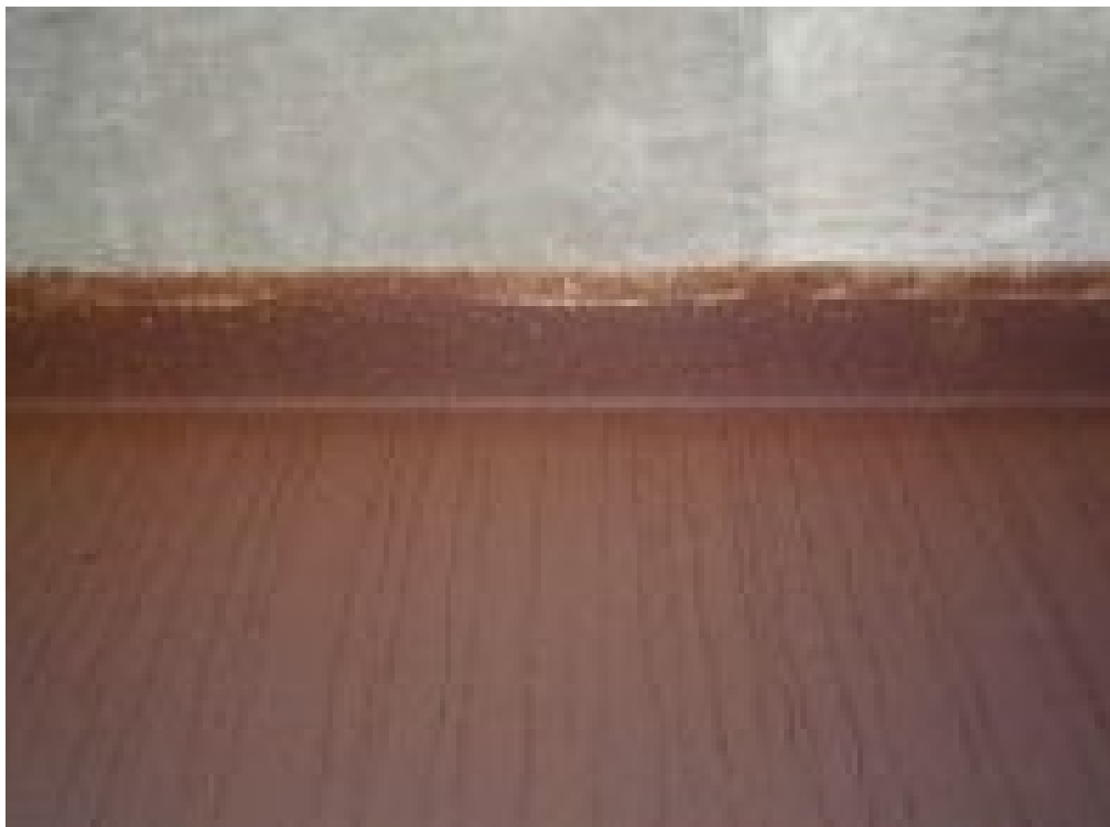
Figure 15 – View of Good Patina with Vertical Variations in Color Due to Condensation (Source: NSBA/AISC 2022)
