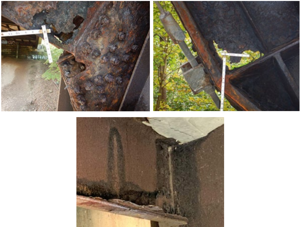
Figure 21 – Advanced Corrosion and Section Loss Due to Leaking Drainage Systems or Leaking Deck Joints
