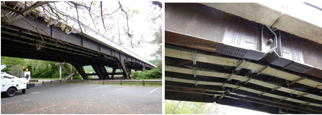
Figure 4 – Views of Multi- Configuration UWS Bridge and Rebuild of Girder at Pinned Joint
