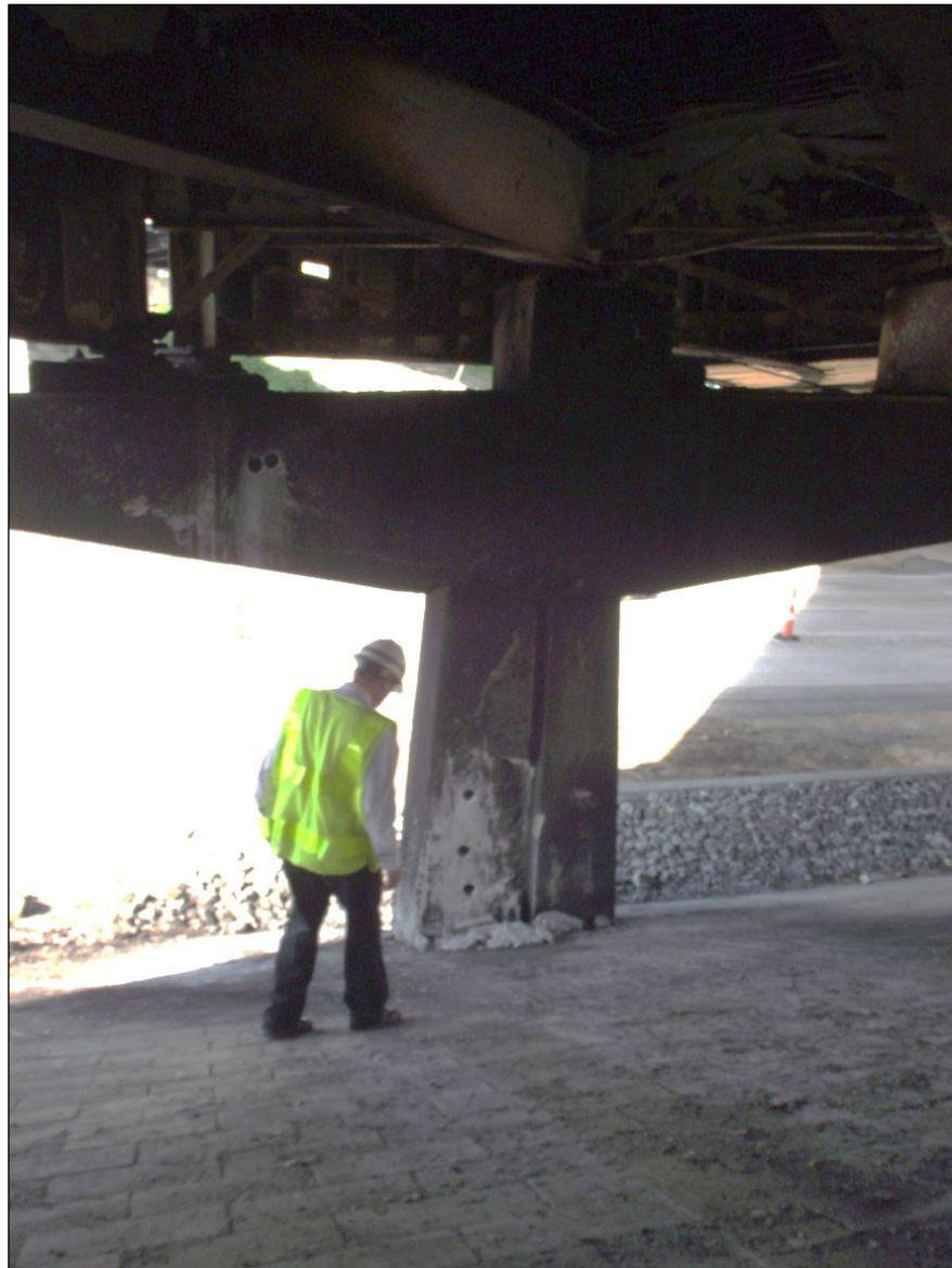
Figure 5 – Location of Concrete Cores
