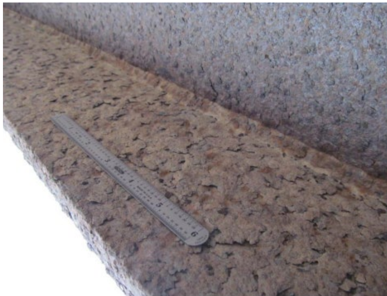
Figure 6 - Large, Thick Loose Flakes Covering the Entire Flange Surface (Source: Crampton et al., 2013)
