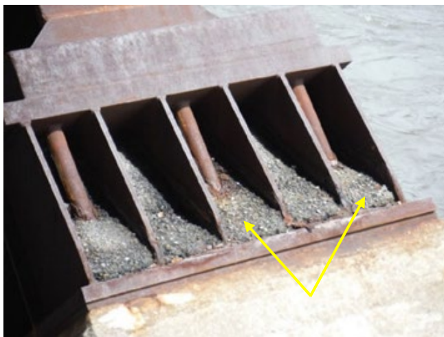
Figure 19 – Bearing Anchorage of UWS Frame Bridge: Views of Ineffective Asphalt Filling and Effective Watertight Steel Panel Retrofit
