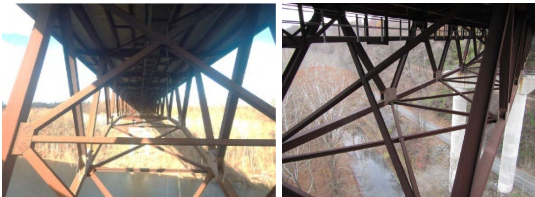
Figure 3 – UWS Deck Truss Bridge
