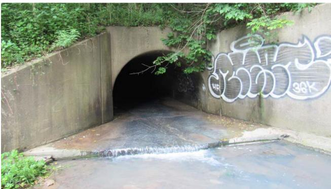
Structure Type 34: Pipe Culvert
