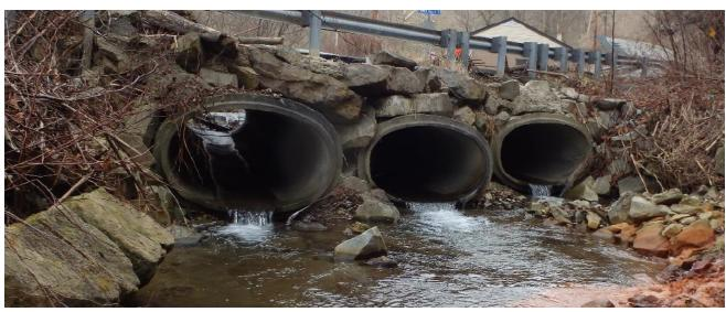
Structure Type 35: Pipe-Arch Culvert
