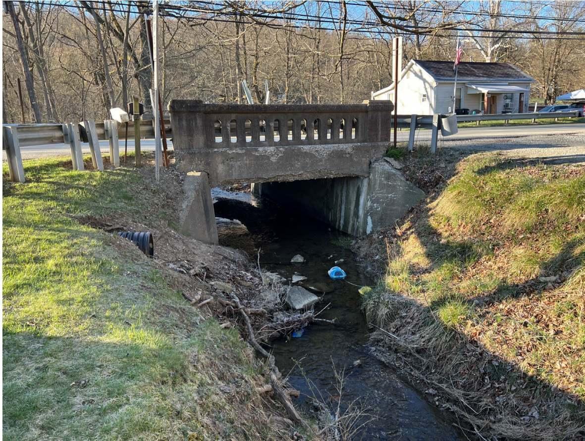
Standing Upstream Looking Downstream
