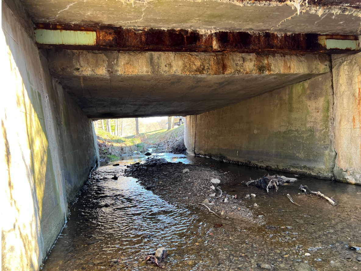
General Underside View
