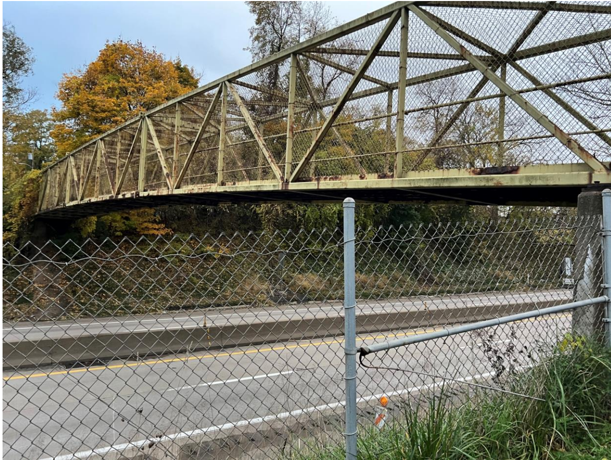
EXISTING PEDESTRIAN BRIDGE VIEW LOOKING SOUTHWEST
