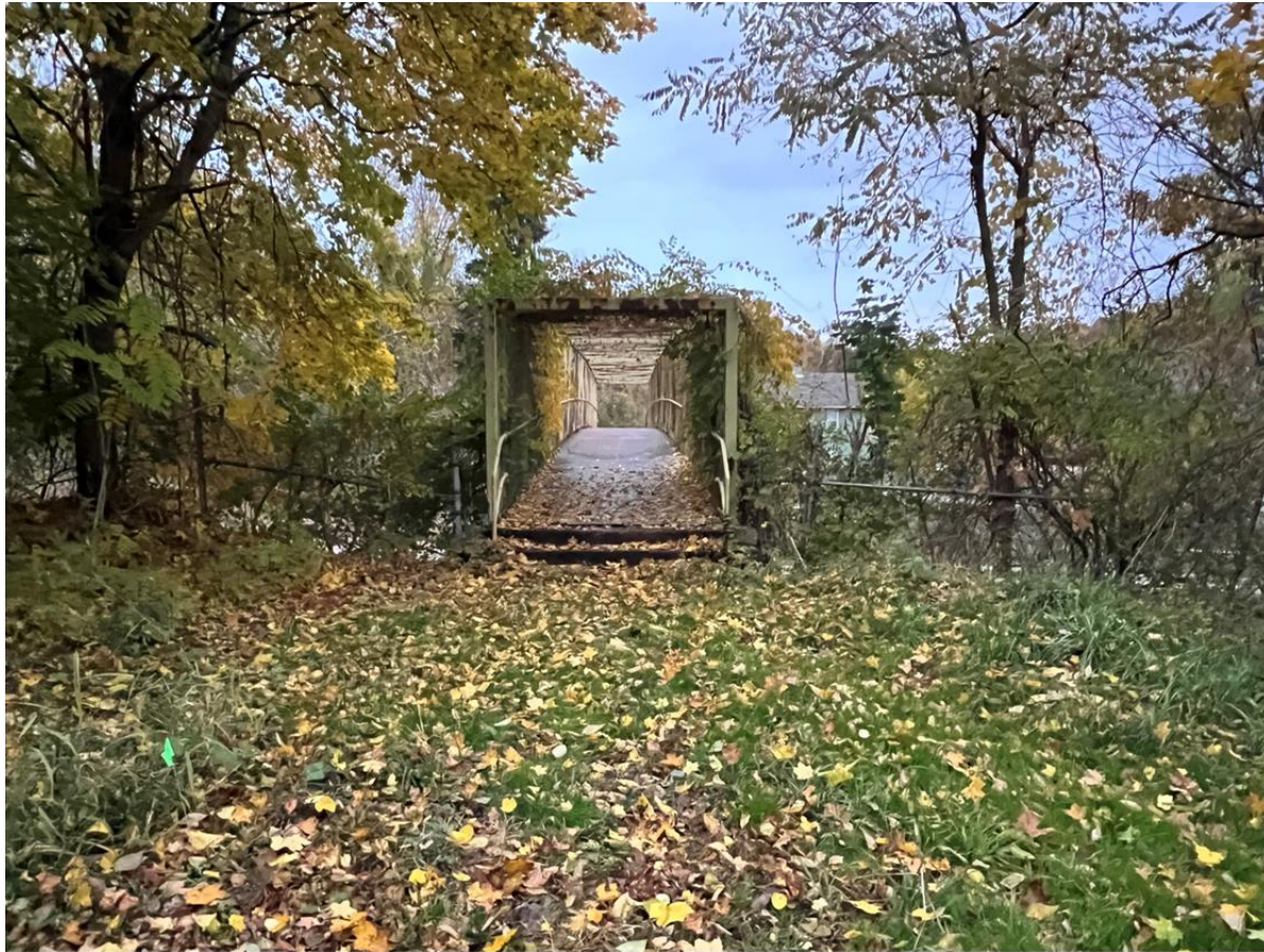
EXISTING PEDESTRIAN BRIDGE VIEW LOOKING NORTHWEST
