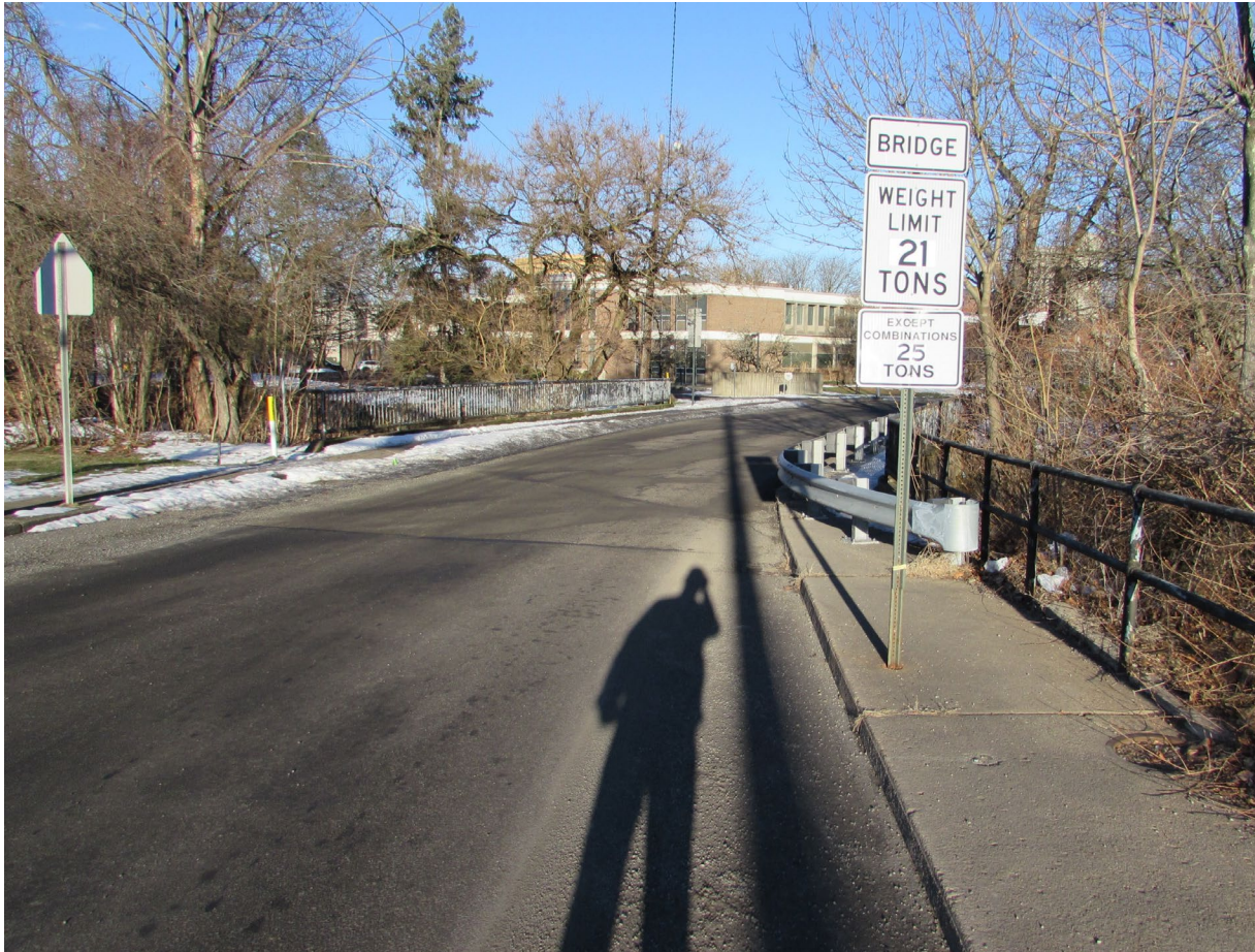
Bridge Southern Approach
