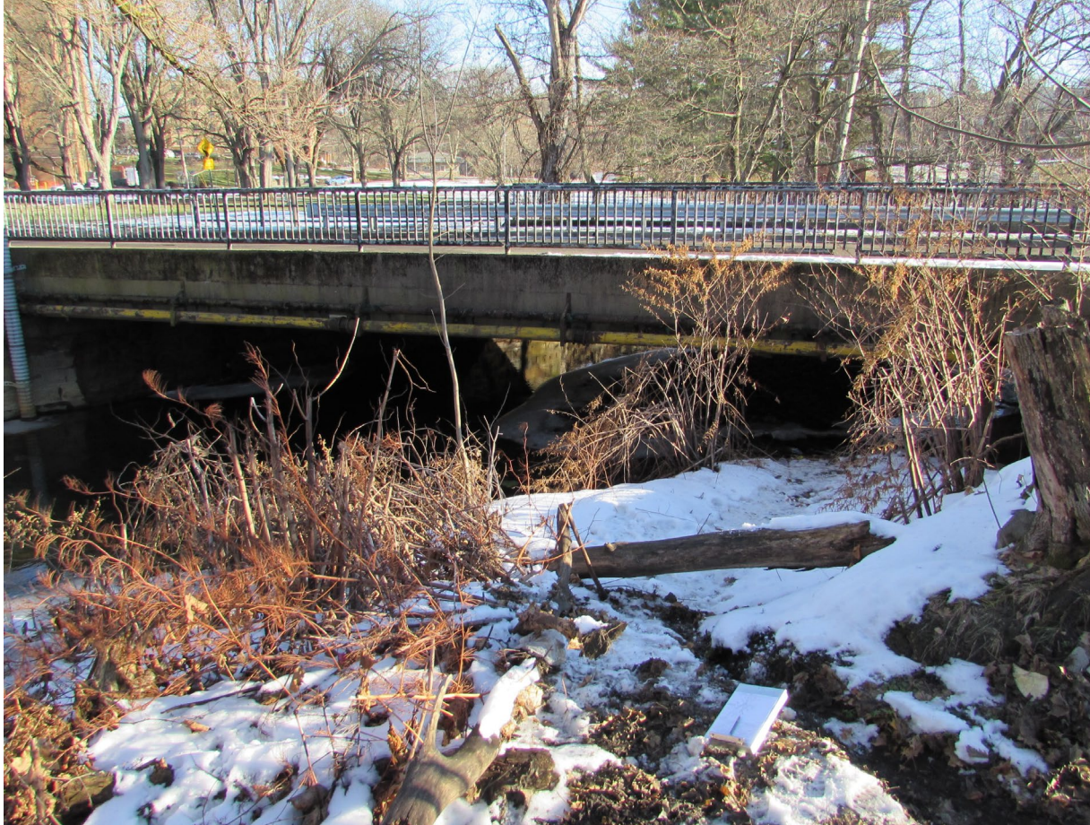
Upstream of Bridge
