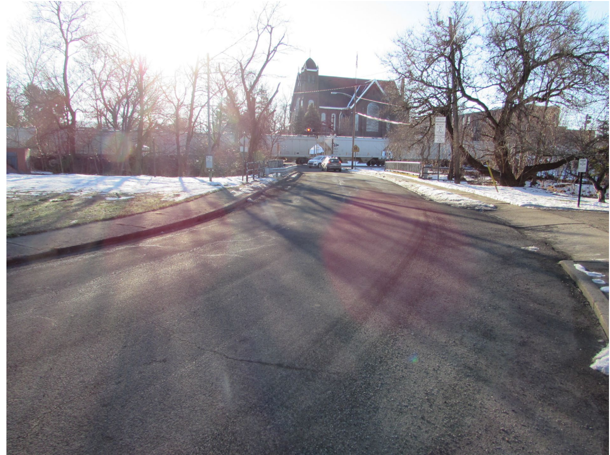
Bridge Northern Approach
