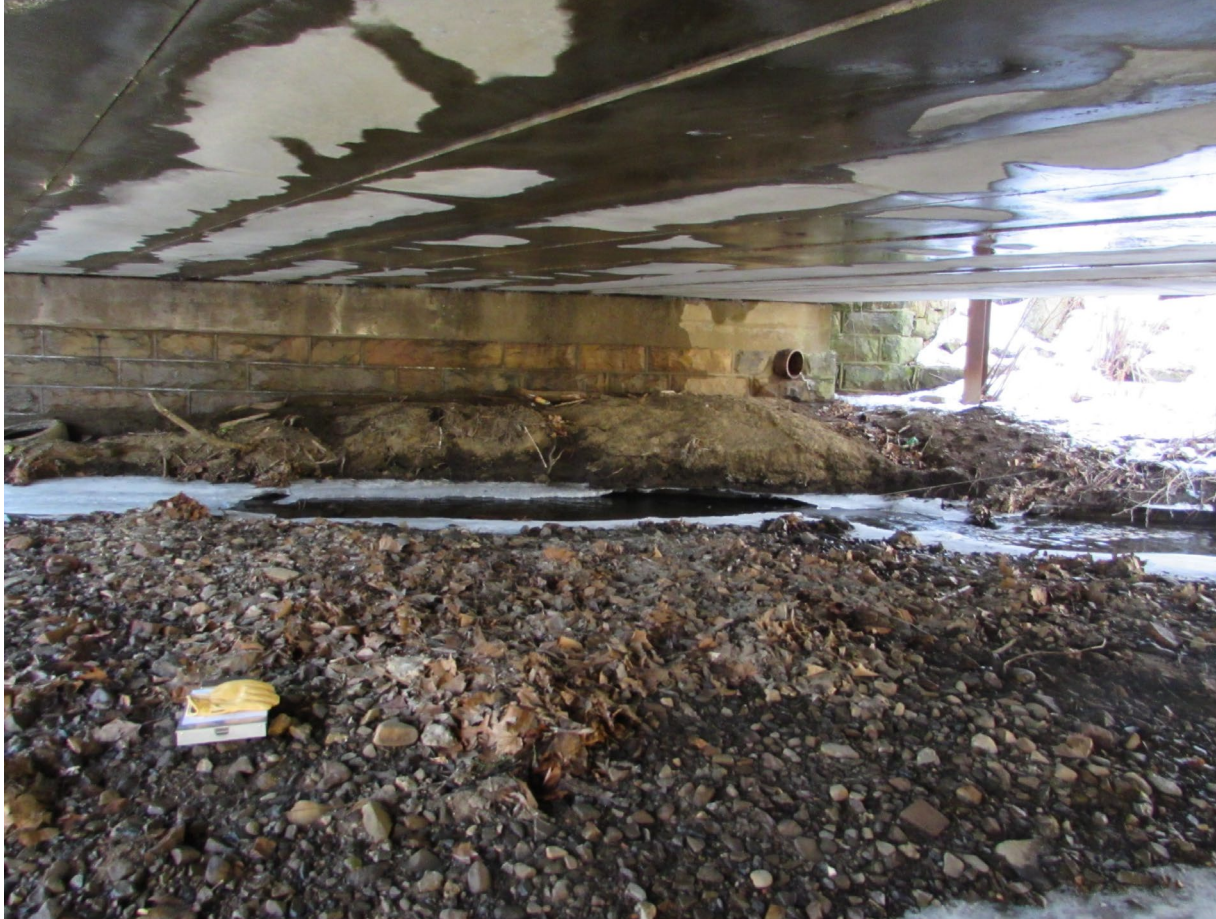
Below Bridge Looking North
