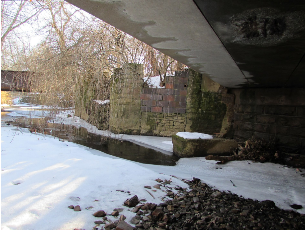
Downstream Retaining Wall
