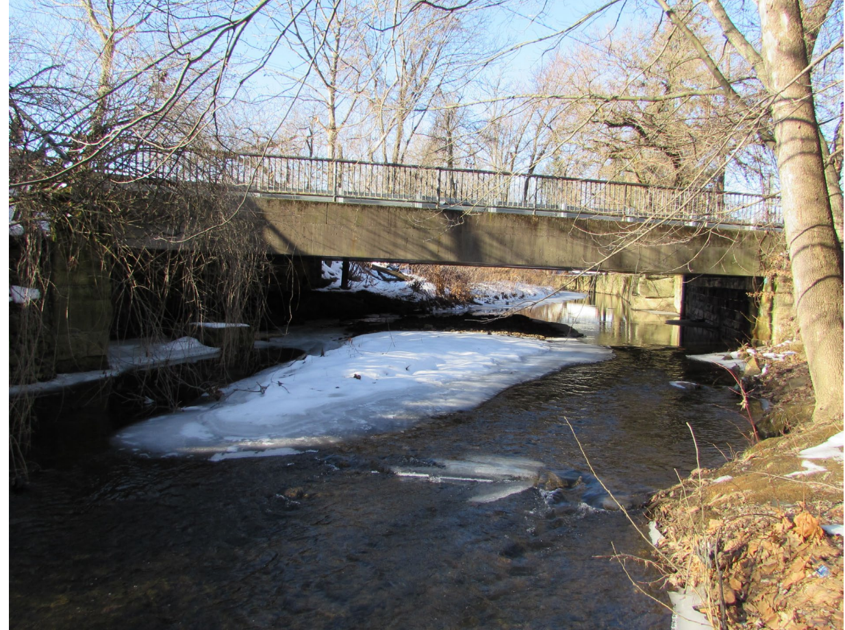
Downstream of Bridge
