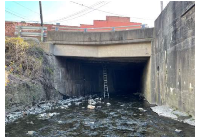
Lincoln Avenue Bridge #13
