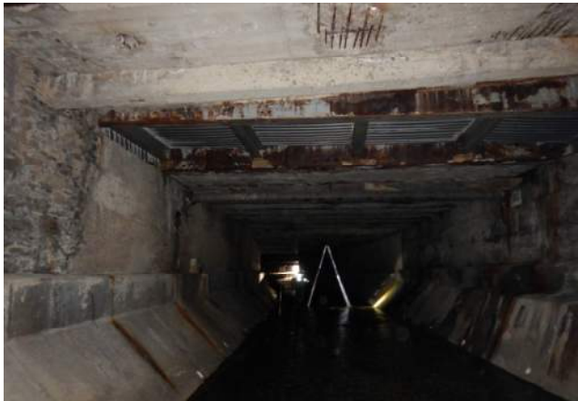
Lincoln Avenue Bridge #7
