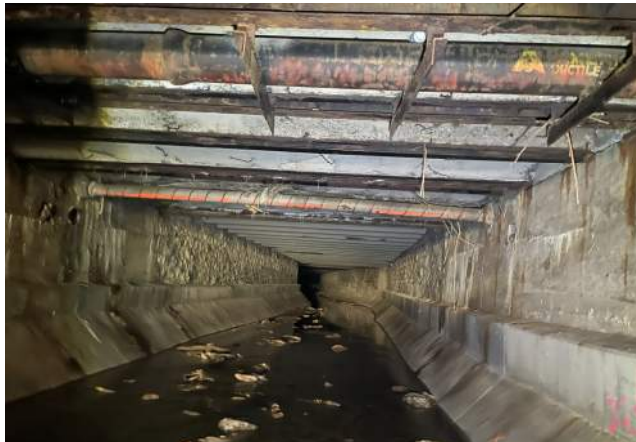
Grant Avenue Bridge #8
