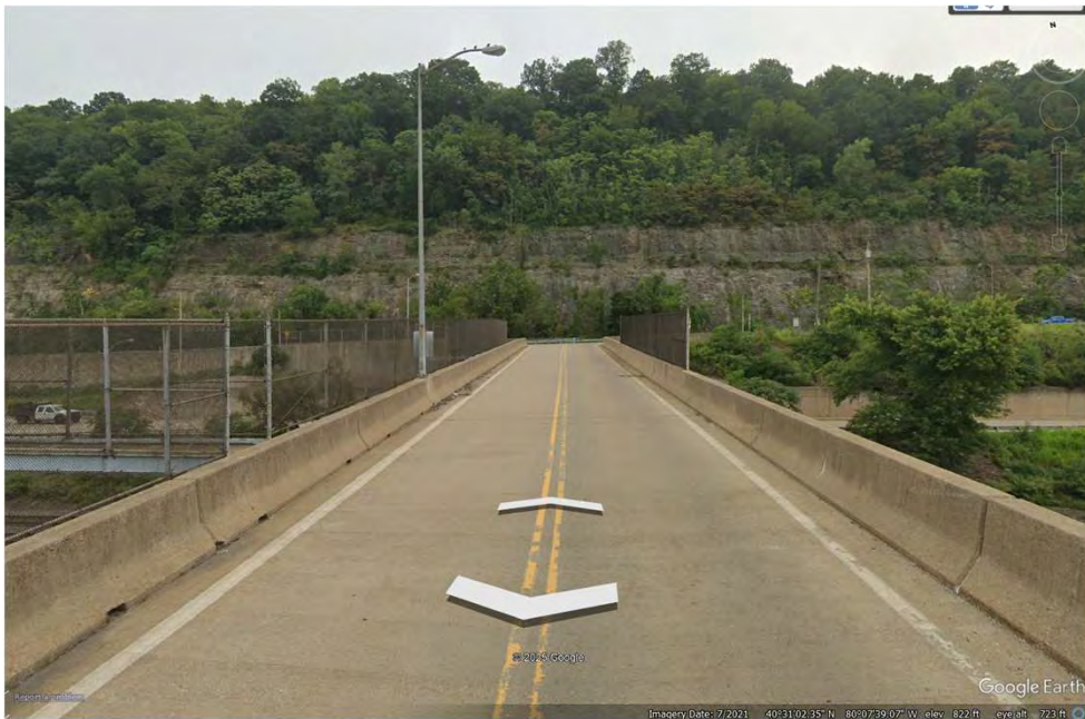
Narrow Bridge Deck
