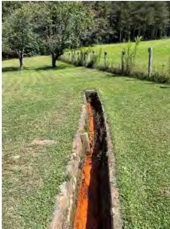
Photograph 21: Unplugged Artesian Well, Alignment DU/E, Station 2403±, Offset 1250±' LT
