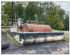
10. View of the 6,000-gallon diesel AST and containment dike with surrounding staining located on the Orner & Sons Trucking property.
