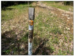
18. View of a typical gas pipeline marker observed within both Segment 2 DU and Segment 2 E, 0.01 miles north of the Mason and Dixon Line.
