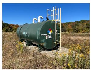
39. View of an aboveground storage tank labeled as containing Caustic Soda near the water treatment pond north of Segment 2 E.
