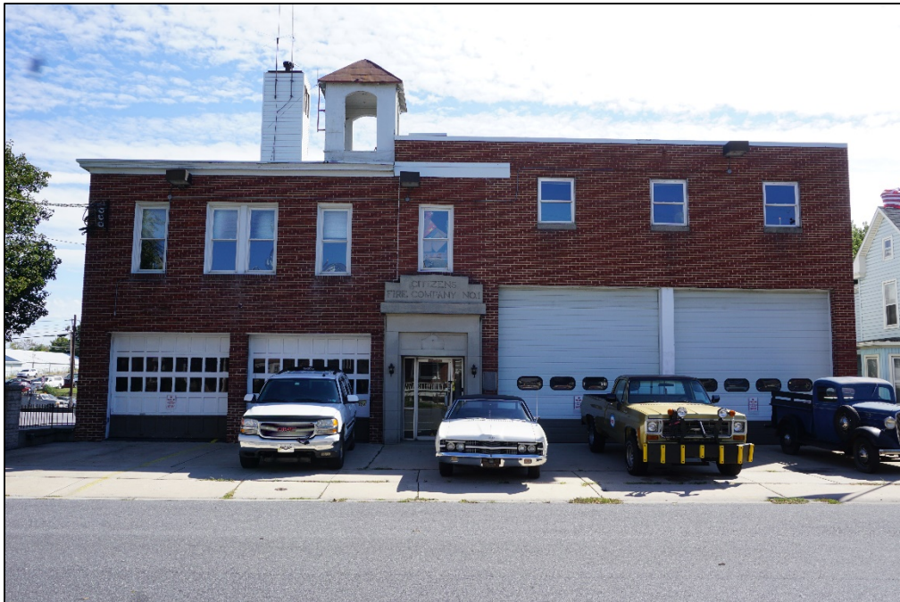
Photograph 11. Northwest (façade) elevation of Citizens Fire Company No. 1, facing southeast.
