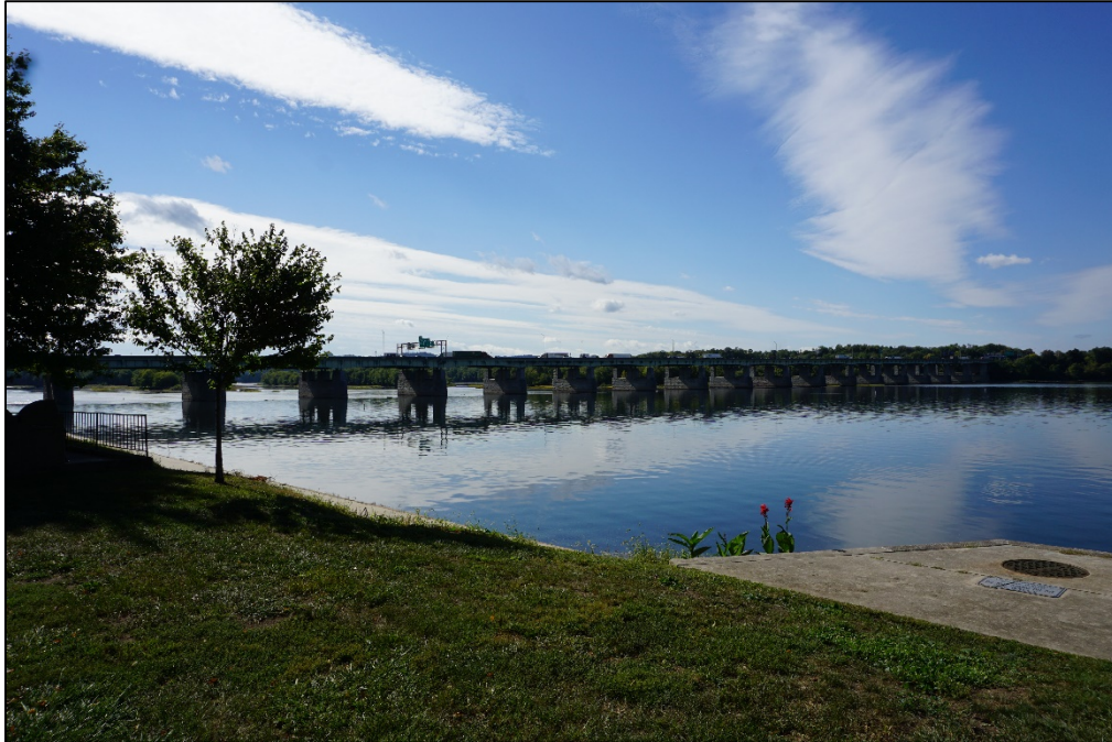
Photograph 1. View of the John Harris Memorial (South) Bridge carrying traffic over the Susquehanna River, facing south.
