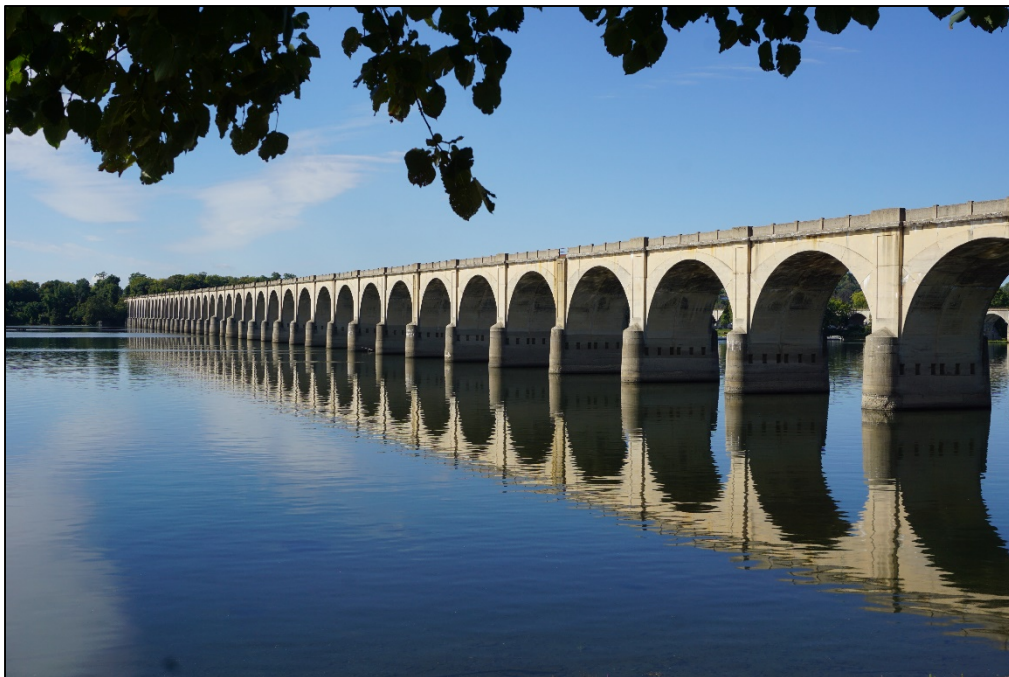
Photograph 28. View of the closed spandrel arch bridge carrying the former Philadelphia & Reading Railroad over the Susquehanna River, facing southwest.
