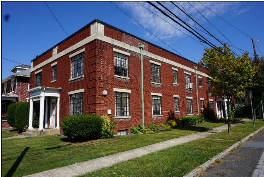
Photograph 21. Southwest (façade) and southeast (side) elevations of the apartment building at 450 S. 3 rd Street, facing north.
