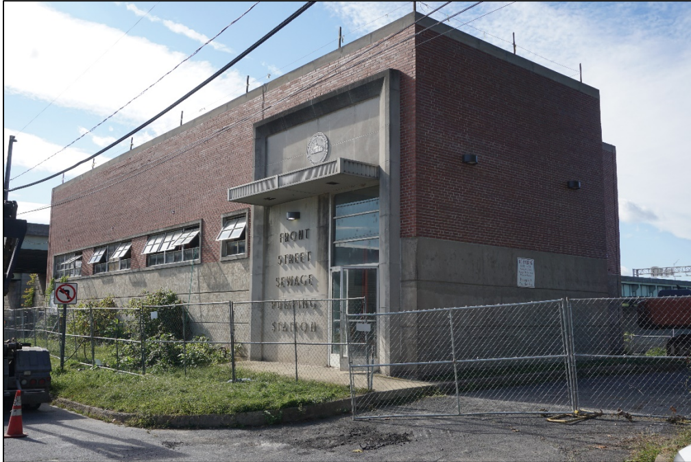
Photograph 30. View of the east and north elevations of the Front Street Sewage Pumping Station, facing south.
