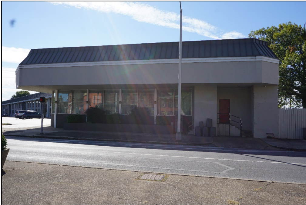
Photograph 29. View of the office of the Quality Inn/Passage to India, facing south.
