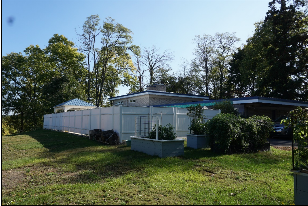
Photograph 23: View of the northwest elevation of the property at 83 Carol Place, facing northeast.
