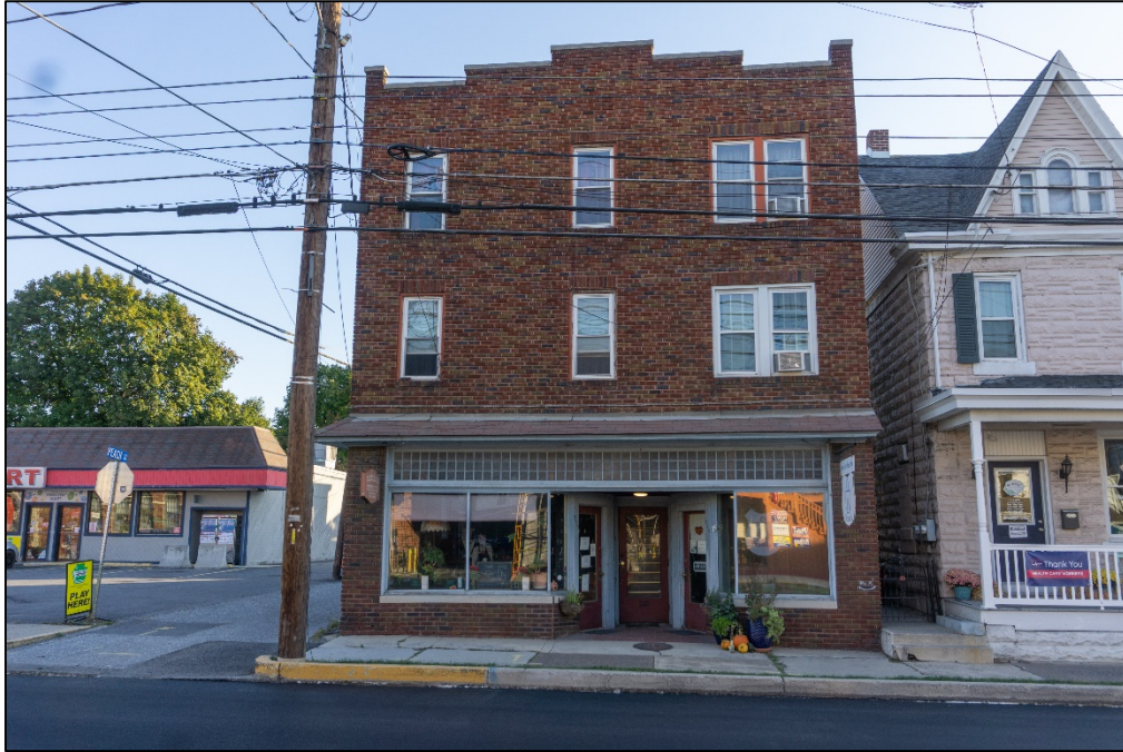
Photograph 14. Southwest (façade) elevation of the Jacob A. Kunkel Building, facing northeast.
