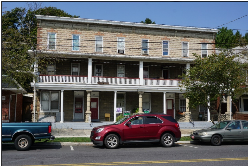
Photograph 17. Southeast (façade) elevation of the S. B. Leach Apartment building at 235-241 Hummel Avenue, facing northwest.
