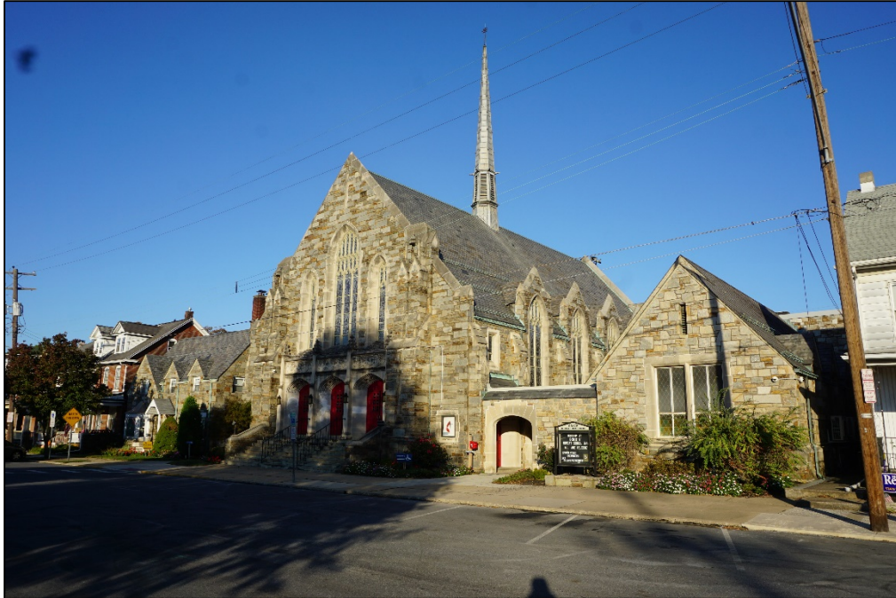
Photograph 12. Southeast (façade) elevation of Grace United Evangelical Church, facing northwest.
