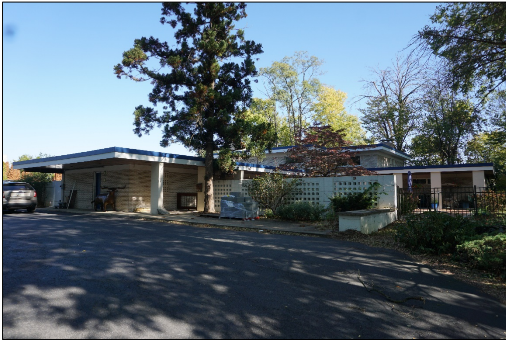
Photograph 22. View of the southwest elevation of the property at 83 Carol Place, facing north.
