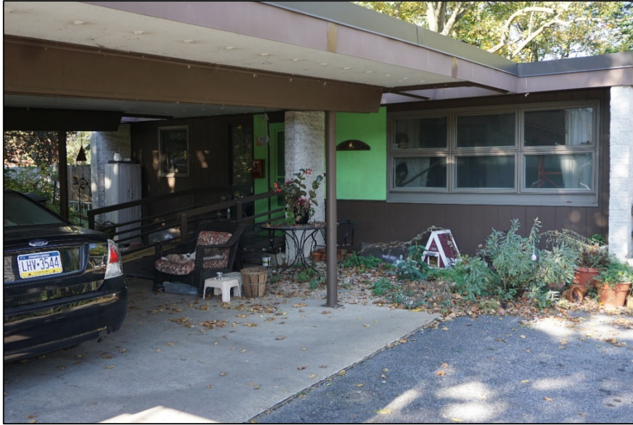
Photograph 20. Southeast (façade) elevation of 347 Lowther Street, facing west. Note the features of the Mid-century Modern style like the projecting wall sections and shallow-pitched roof with a large attached carport.
