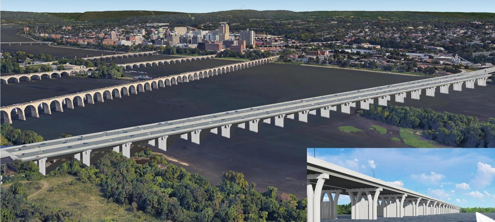
This rendering of what the potential replacement South Bridge could look like is based on a multi-girder bridge design. The exact bridge type will be selected during final design.
