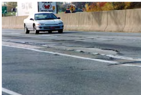
[1] Deteriorated Pavement
