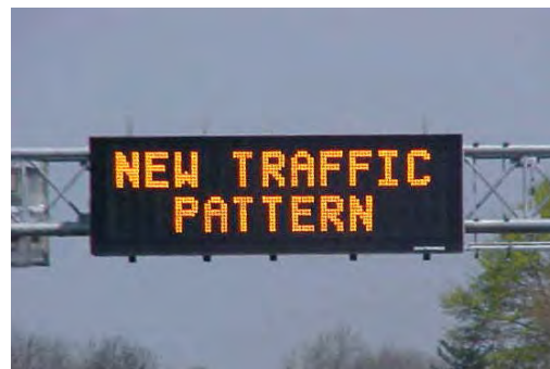
One of the existing variable message signs on I-83, an ITS application
