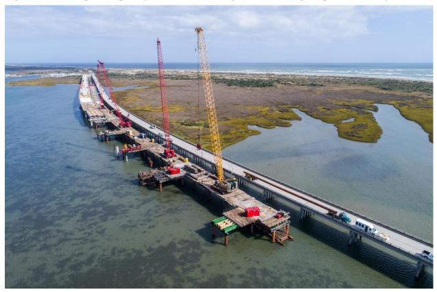
Figure 2-12. Example Temporary Construction Bridge (Bonner Bridge Replacement Project, HDR)
