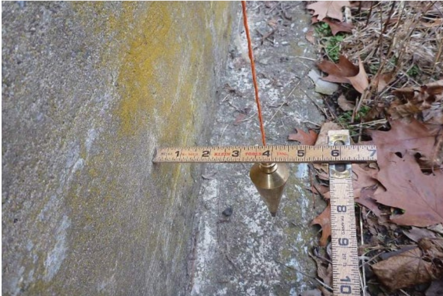
Photo showing area of wall that is leaning
