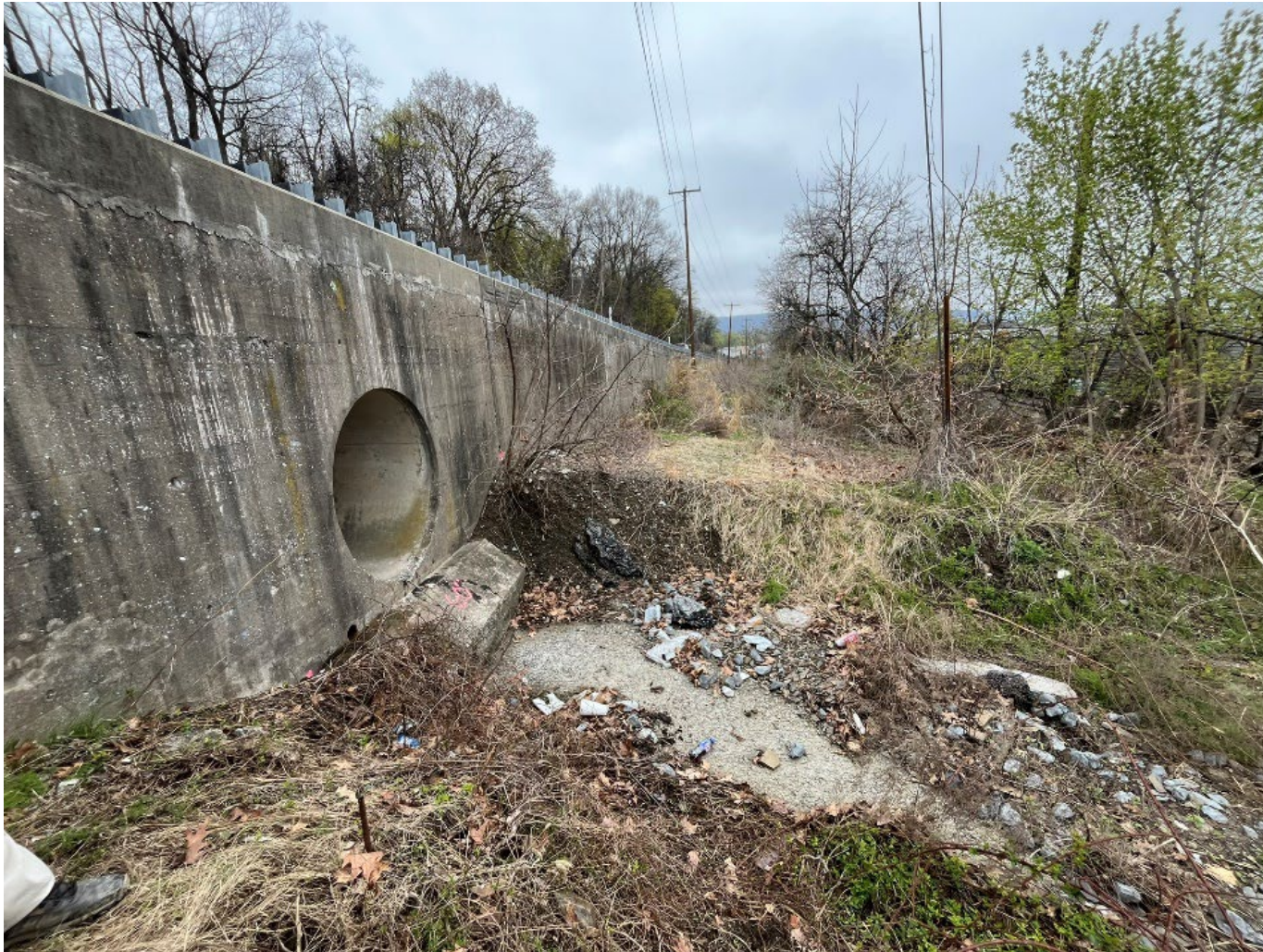
Drainage Pipe through wall near the middle section of the wall
