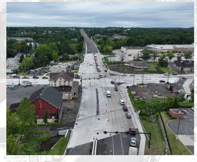
Both of the precast box culverts on Skippack Pike have been installed and the contractor has completed the construction of the cast in place wing walls, distribution slab and approach slabs at the culvert on the west leg of Skippack Pike.
